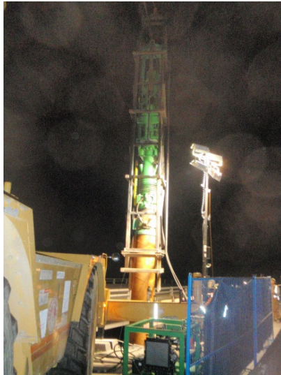
Figure 9 – Pile Driving at Night
