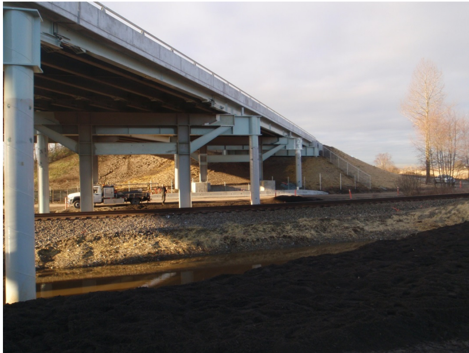
Figure 11 – Retrofit of Existing Pier Support
