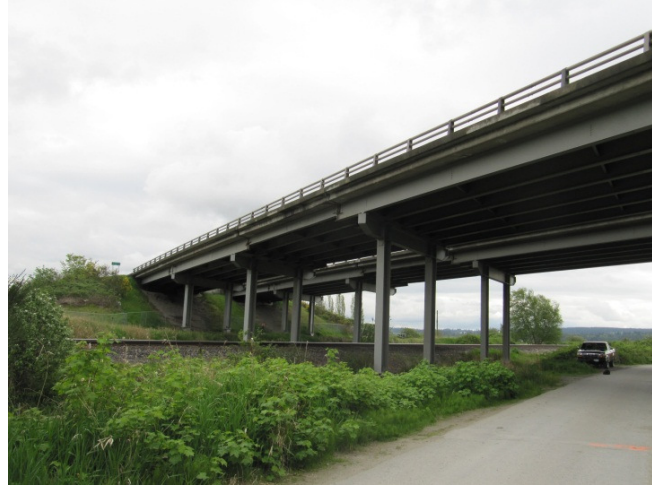
Figure 2 – Existing Bridge Structure
