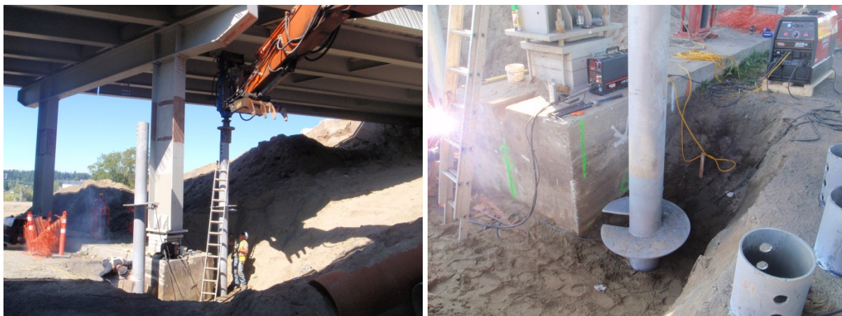
Figure 10 – Driving of the Helical Piles
