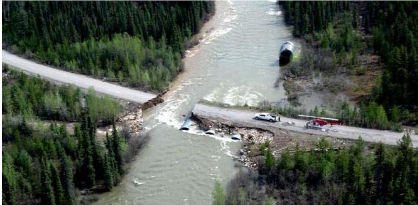
Figure 1: The Nahanni Range Road, which leads to the mine, was washed out in three locations. (Yukon Department of Highways and Public Works)
