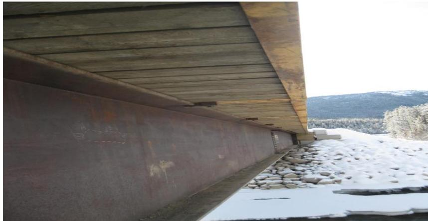
Figure 14: Underside view of girder and deck after permanent placement
