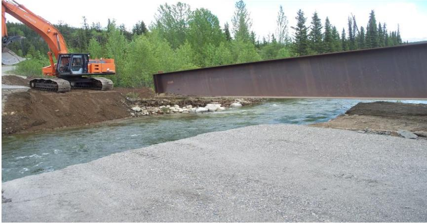
Figure 5: A view of girder launching
