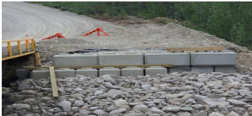
Figure 12: Half of permanent abutment
