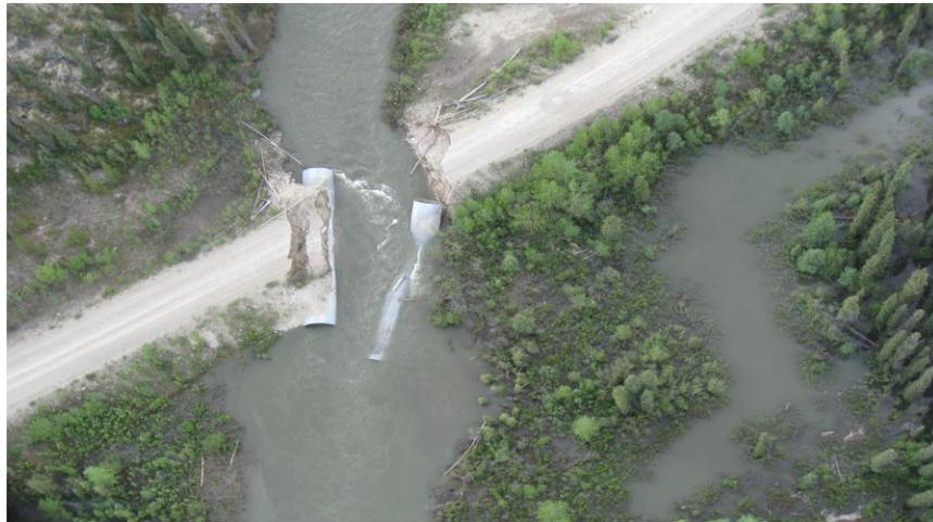
Figure 3: Aerial View of Highway#10 after washout Km74
