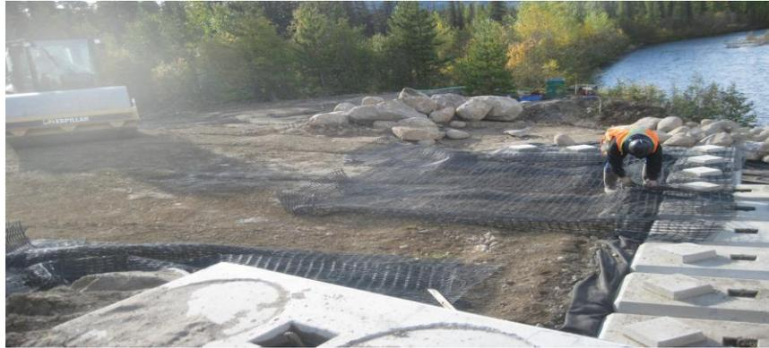
Figure 11: Placing of Geogrid
