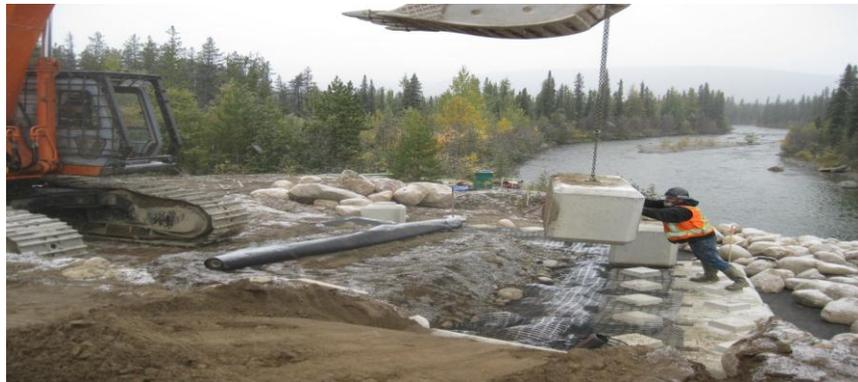
Figure 10: Lowering and placing of lock blocks
