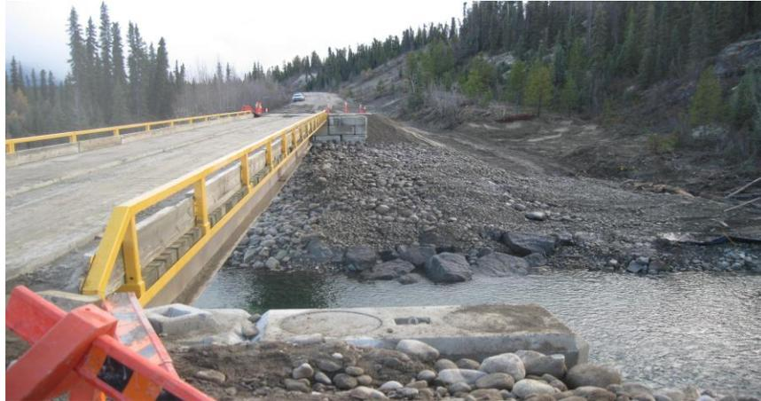
Figure 13: Bridge after placing on lock blocks
