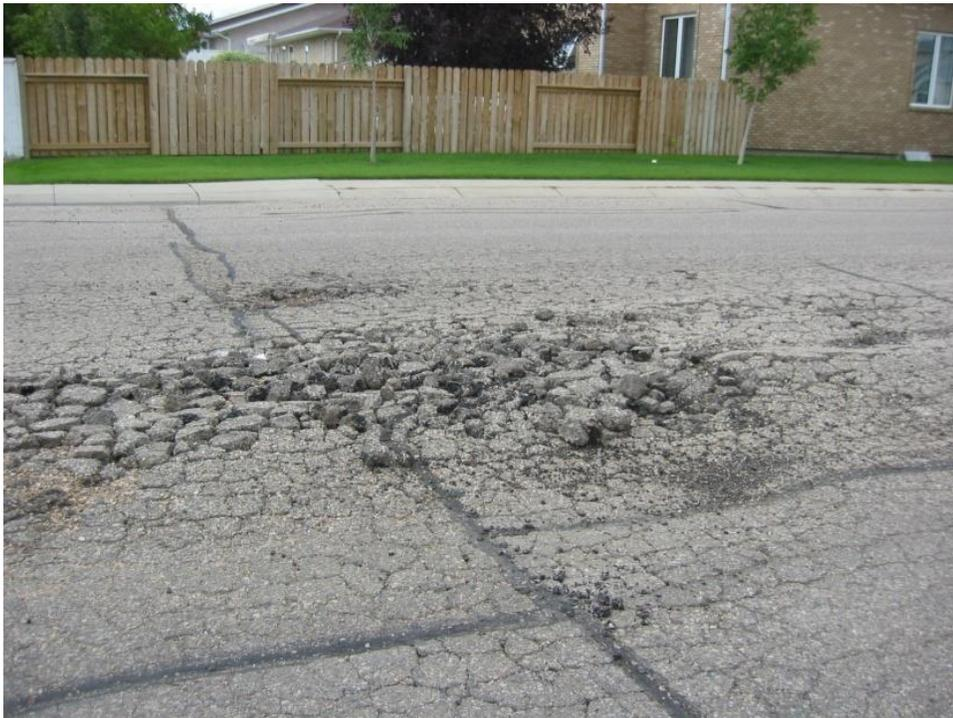
**Figure 2**      **Typical City of Saskatoon Roadway Structural Failure**
