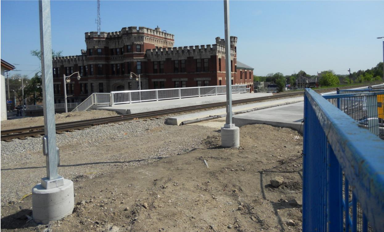
**Photo 16 - Rail Bridge South Track Operational, North Track Ready for Ballast**
