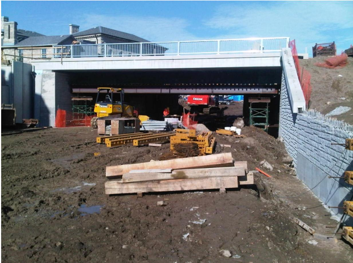
**Photo 11 - MSE Wall and Bridge Structure Shoring**
