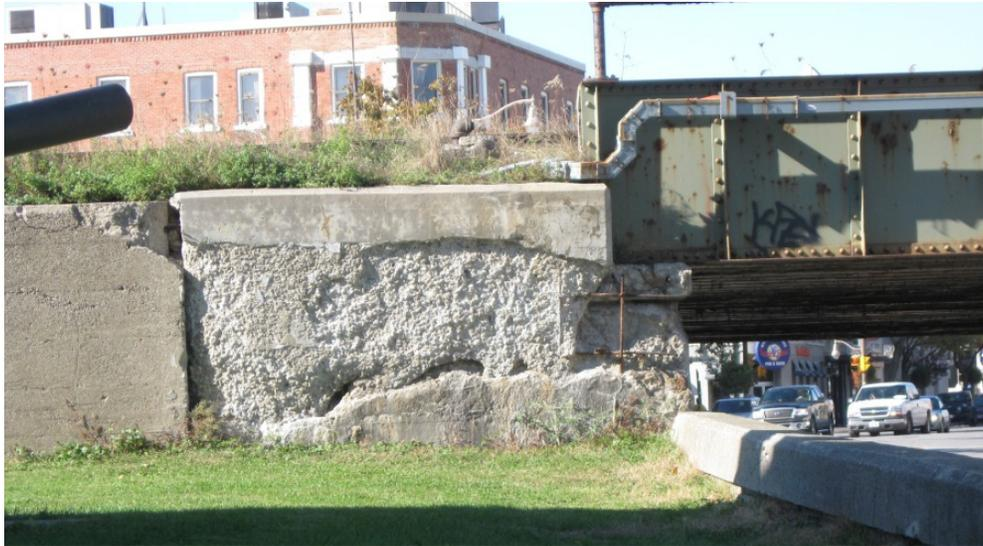
**Photo 4 - South West Retaining Wall and Bearing Seat Deteriorations**
