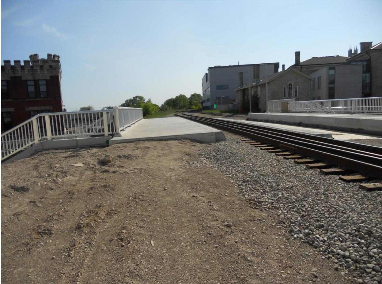
**Photo 14 - Rail Bridge South Track Operational, North Track Ready for Ballast**
