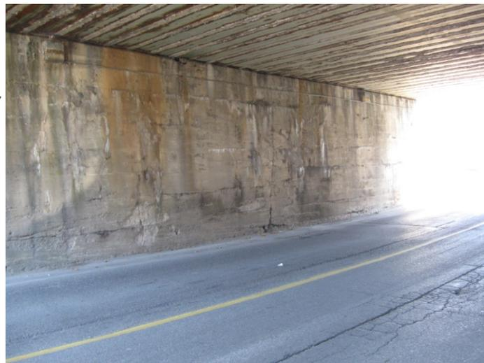
**Photo 6 - East Abutment Wall and Bridge Soffit**
