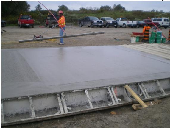
c) Finishing of concrete with bull float and burlap drag
