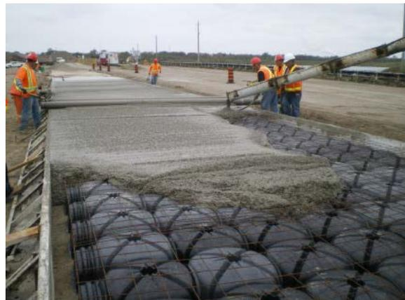
b) Placement and consolidation of concrete
