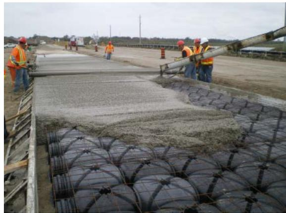
b) Placement and consolidation of concrete
