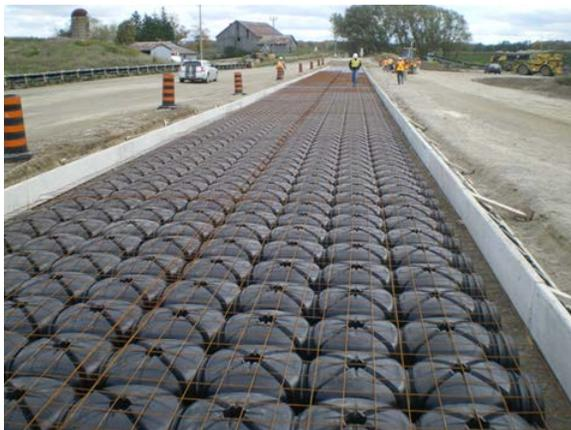
a) Formwork units laid out with wire mesh on top
