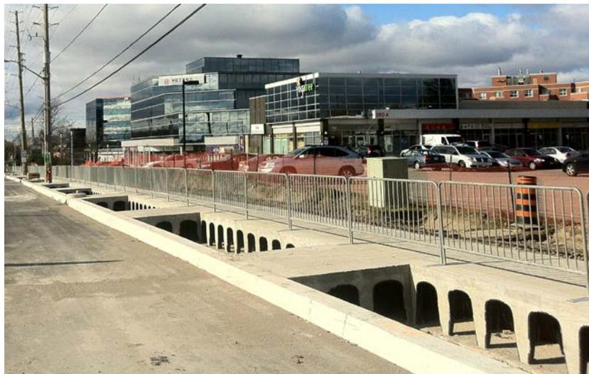
**FIGURE 10 Sidewalks incorporating the dome-shaped formwork system.**
