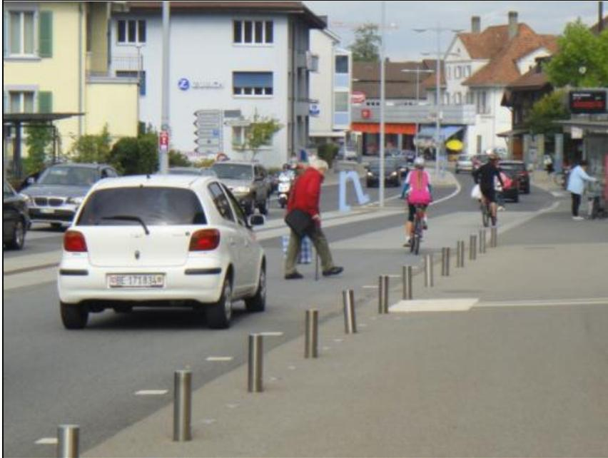
**Figure 8** Crossing in a two-step sequence allows to concentrate on one direction at a time (Köniz, Switzerland)
