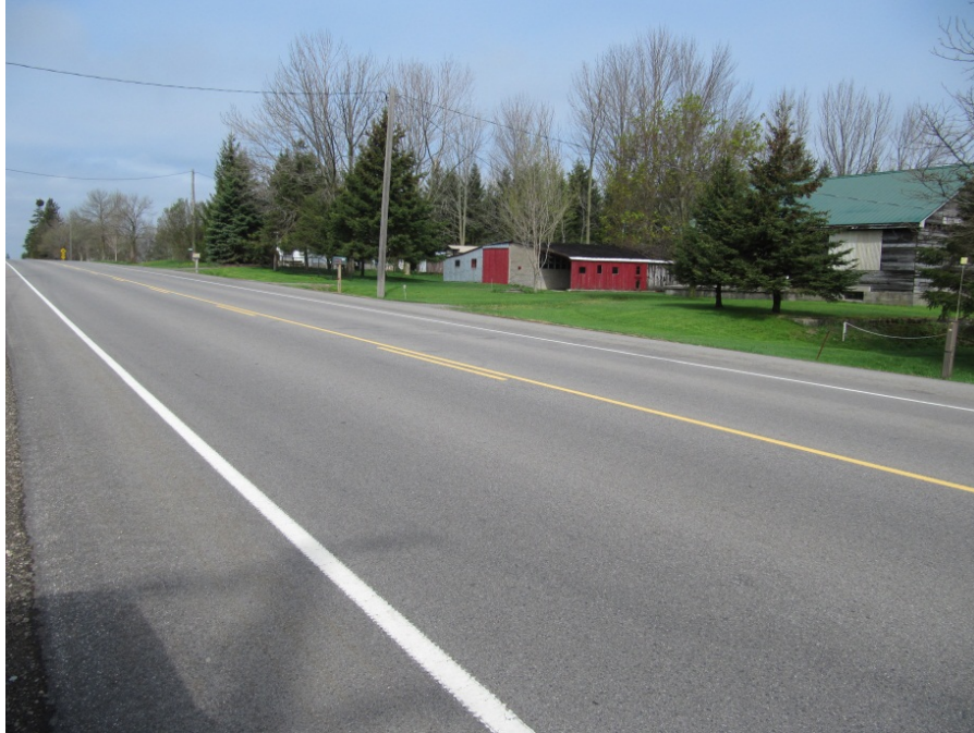
Photograph 8 Excellent condition of new pavement pulverized and asphalt overlaid in 2013 on RR 4.
