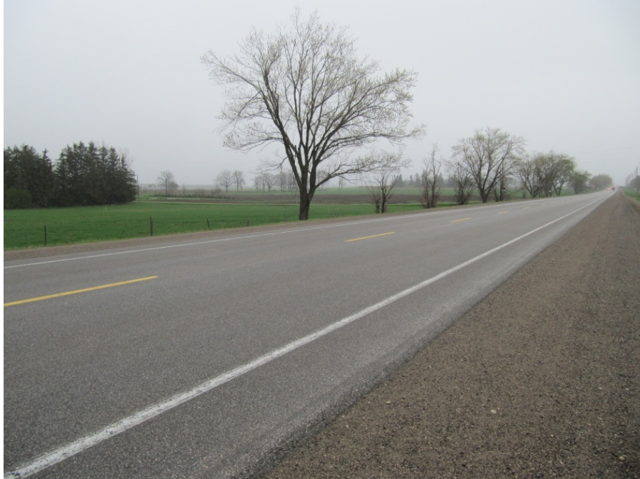
Photograph 7 Very good condition of 5 years old CIREAM stabilized pavement on RR 86.
