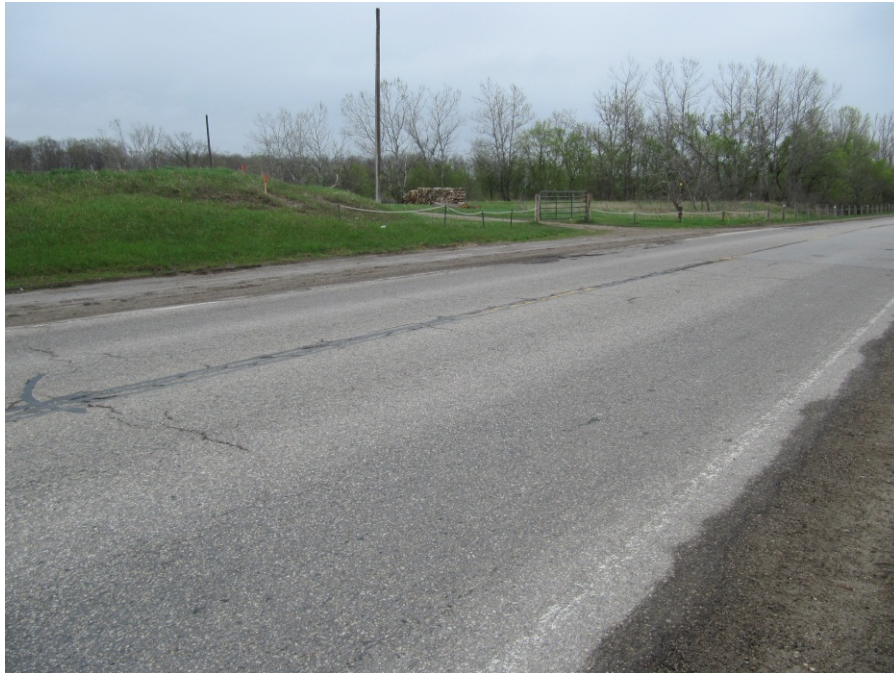
Photograph 1 Joint and transverse cracking on 18 years old Cold In-place Recycled pavement on RR 16.
