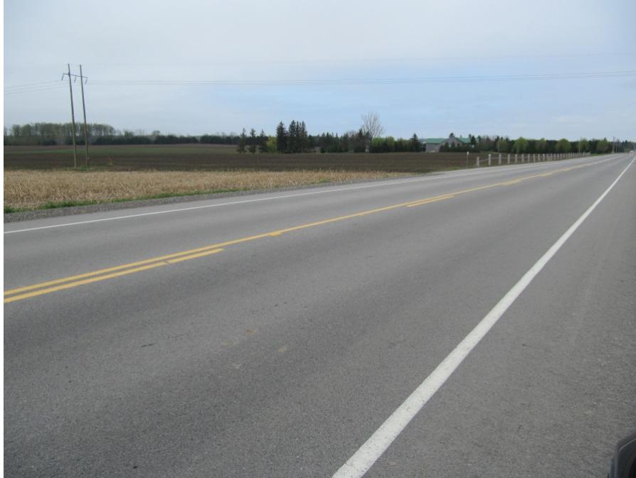
Photograph 10 Excellent pavement condition of a section of RR 4 after application of thin asphalt overlay in 2013.
