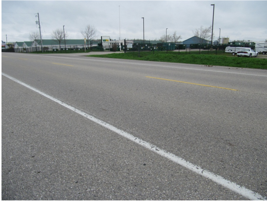
Photograph 2 Good current condition of 10 years old Cold In-place Recycled pavement on RR 15 section between Three Bridges and RR 8.
