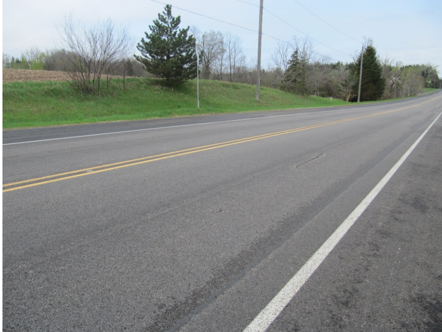
Photograph 9 Some of the cracks in the underlying asphalt pavement have reflected through the bonded wearing course after one winter on RR 4.
