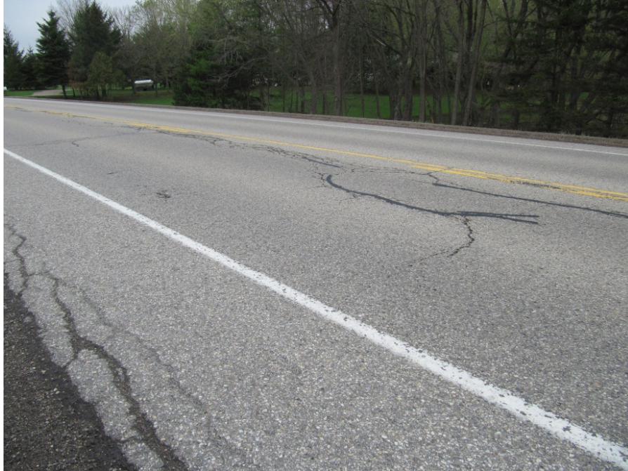
Photograph 3 Centerline, edge and localized alligator cracking in 19 years old pavement on RR 15 section from Martin Creek Road to East Limit of Heidelberg.
