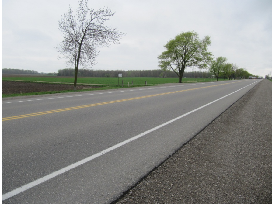
Photograph 5 Excellent current condition of 4 years old foamed asphalt stabilized pavement on RR 8.
