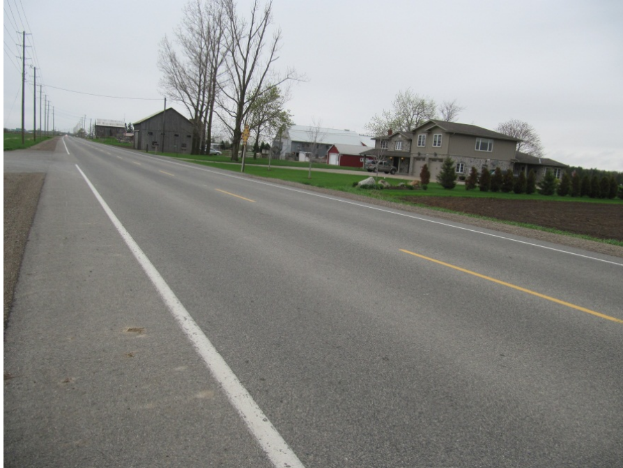
Photograph 4 Excellent current condition of 5 years old re-recycled with foamed asphalt stabilization pavement on RR 22.
