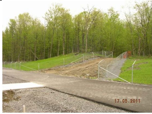
Plate 2. Terminal ends of the fencing at a bike trail opening were wrapped backwards to avoid escapes. Top panels were angled back 45° as some turtles can scale fences using their beak and claws.
