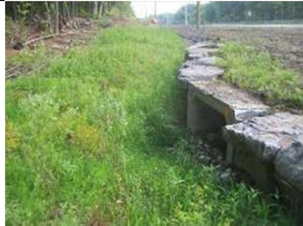
Plate 1. Box culvert with armour stone guide walls on each side. With 30 cm of substrates covering the bottom, the opening is 60 cm tall X 120 cm wide. The 25 cm overhanging lip is meant to stop animals from scaling the walls.
