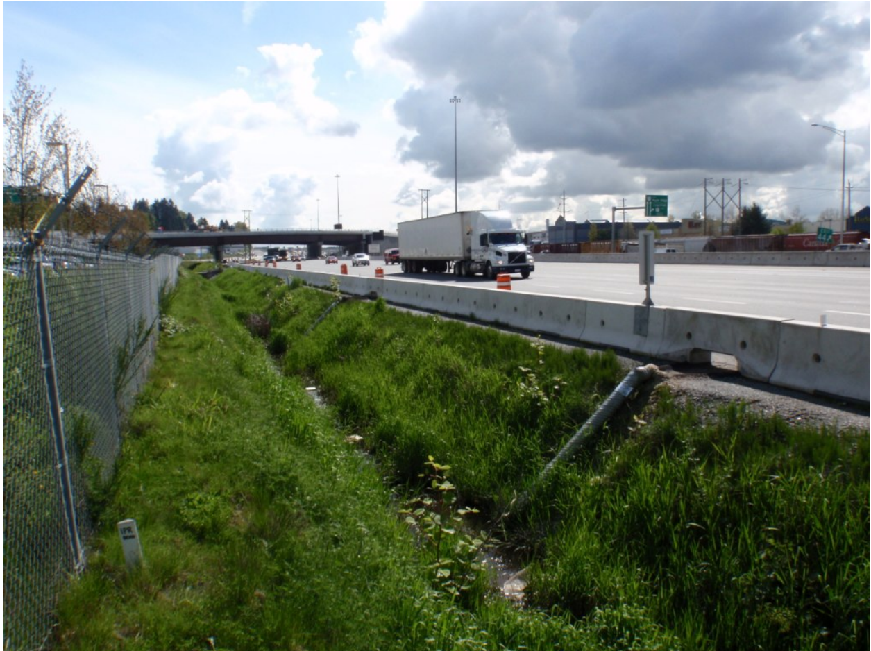
Photo C: RSS at PMH1 Project [Westbound Highway One Lane Widening, April 2014]
