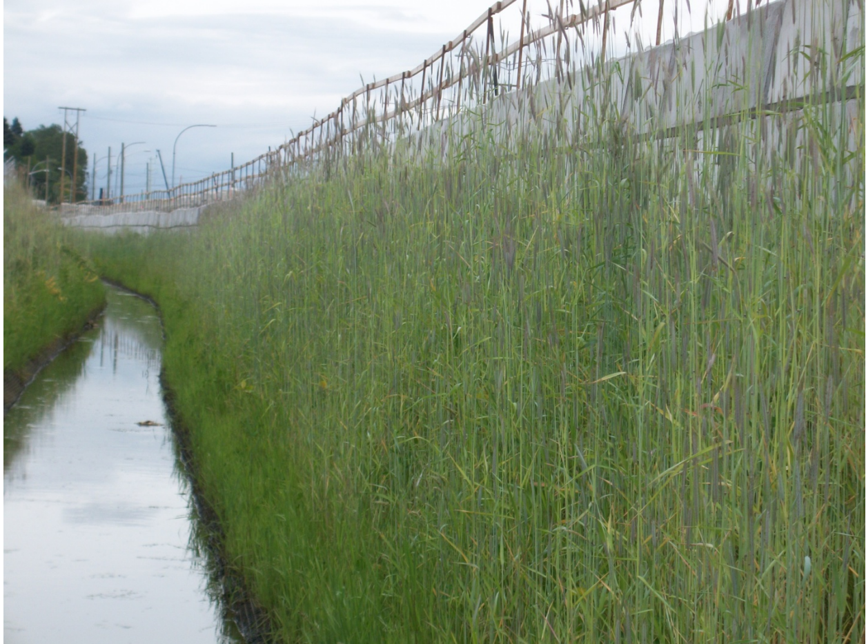
Photo B: RSS at PMH1 Project [Westbound Highway One Lane Widening, May 2010]
