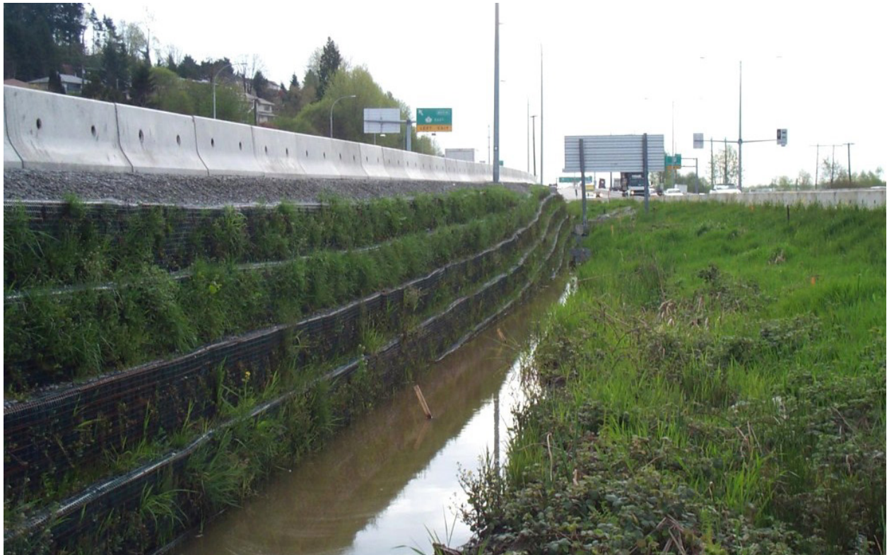
Photo E: Cape Horn I/C at Highway 7[Left Hand Side], and Highway 1[Right Hand Side] [2000]
