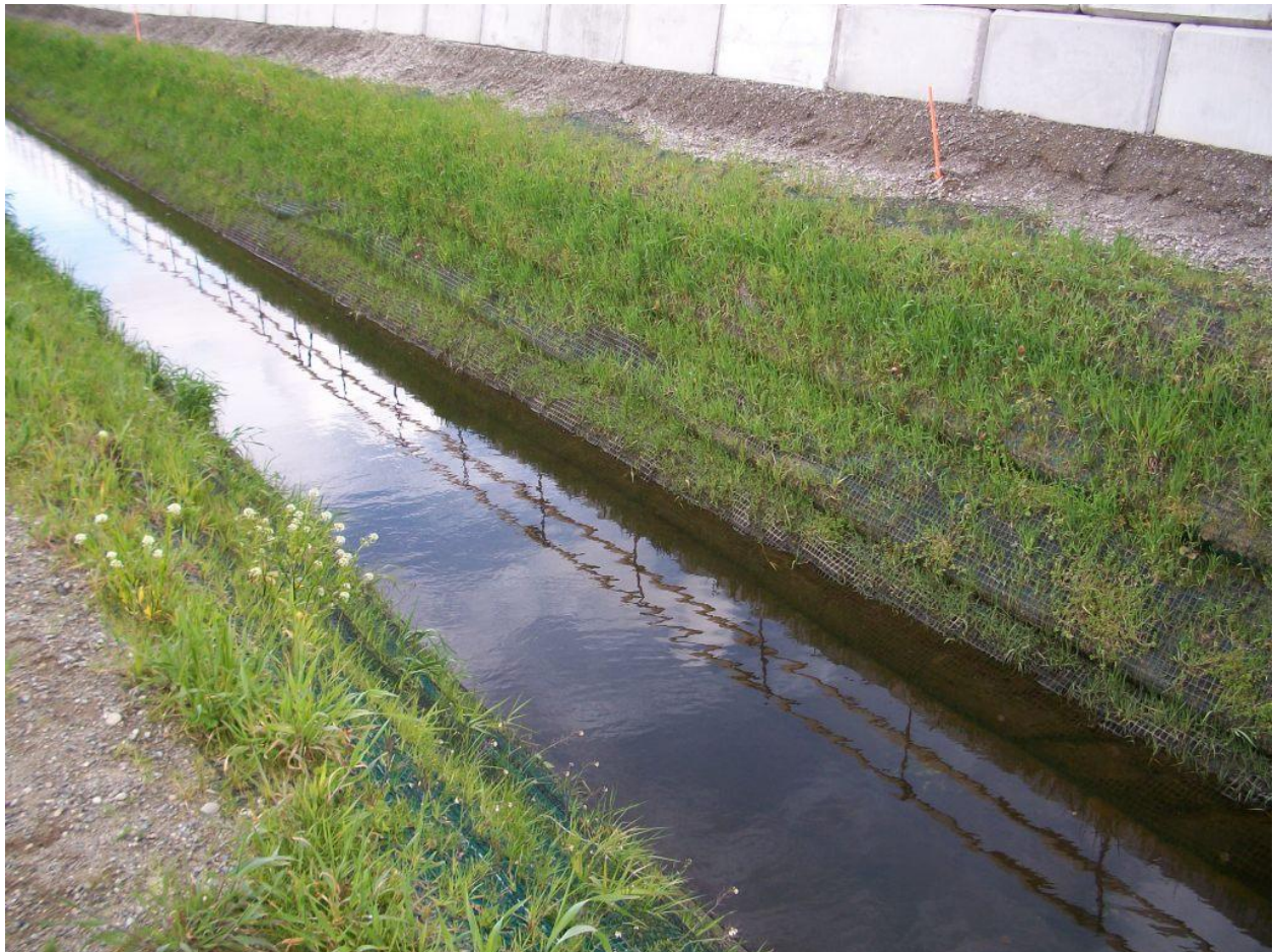
Photo A: RSS at PMH1 Project [Westbound Highway One Lane Widening, April 2010]
