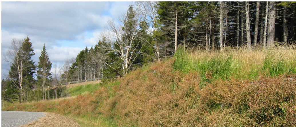
Photo P: Constructed 2009, Fundy National Park Trails, NB, [Photo 2014]
