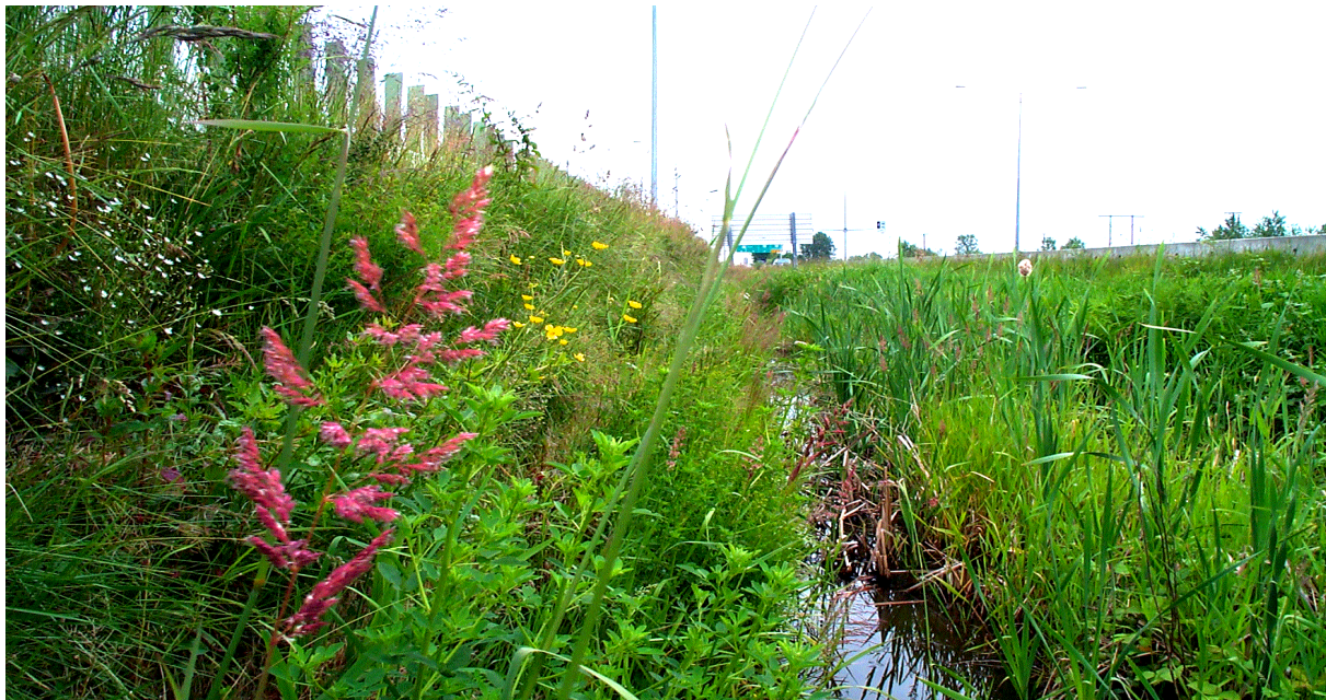
Photo D: Looking Eastbound [Cape Horn I/C along Hwy 7 / 1, Coquitlam, BC Year 2002]
