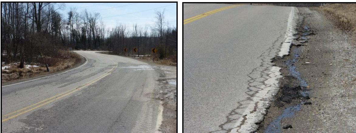
Figure 5: 20 Sideroad edge cracking through curve 2 (eastern curve)
