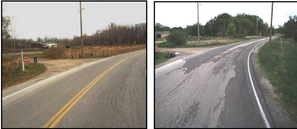
Figure 6: 20 Sideroad pavement conditions through curve 1 (western curve) 2010-left & 2013-right
