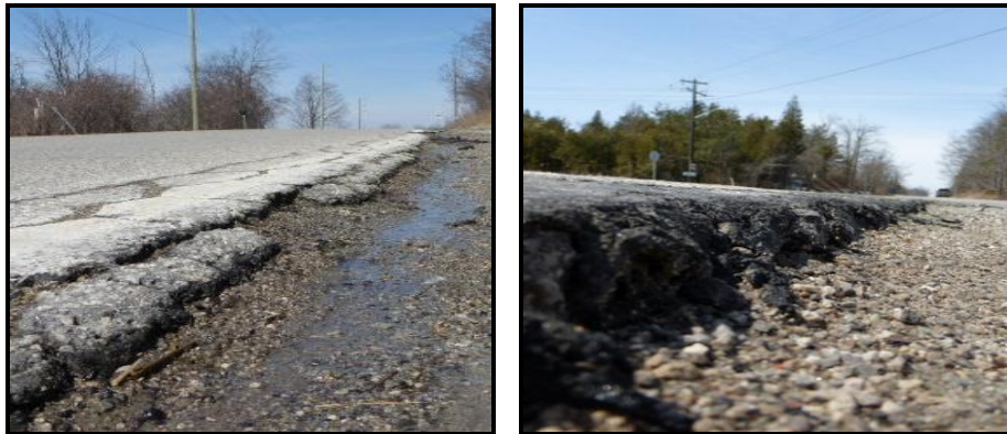
Figure 4: 20 Sideroad typical edges, curve and linear sections
