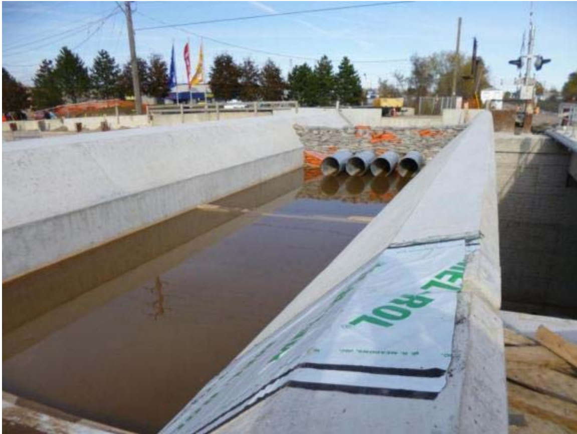
Figure 5 – Indian Creek on structure (temporary connection)
