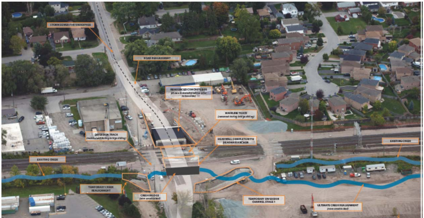
Figure 2 - Underpass structure under construction in place (Background image courtesy of Rocco Cacchiotti)
