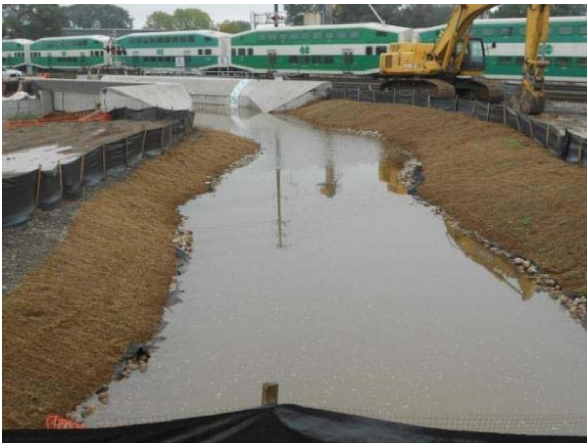
Figure 4 - Temporary interim channel to Creek Bridge
