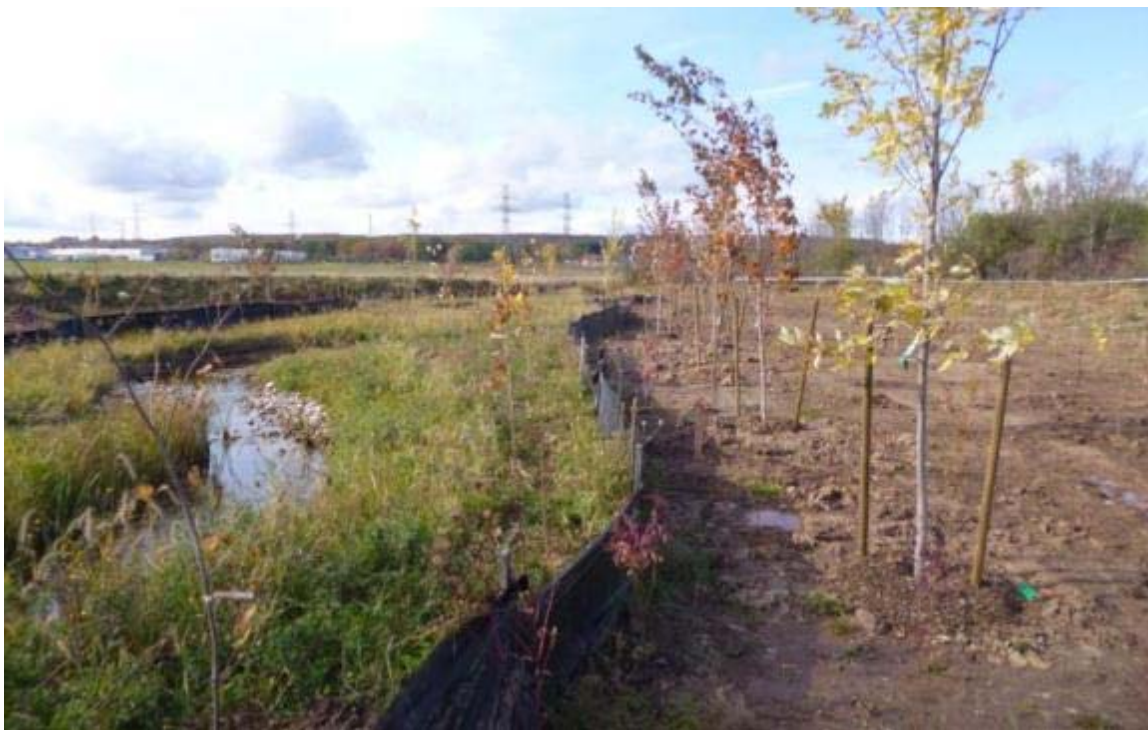
Figure 3 - North/ south creek reach overbanks just planted and thalweg vegetated
