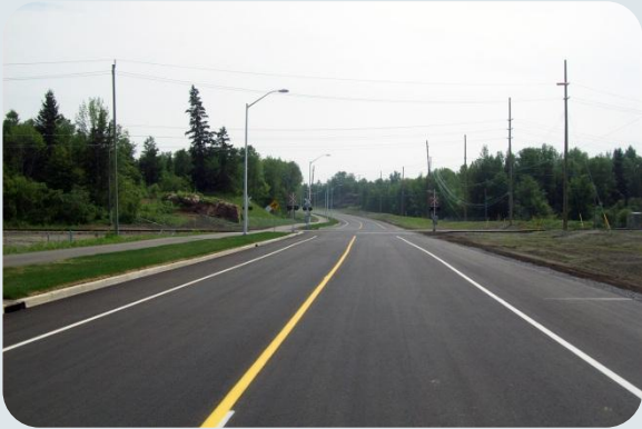
PHOTO 21: Terry Fox Drive – Completed
