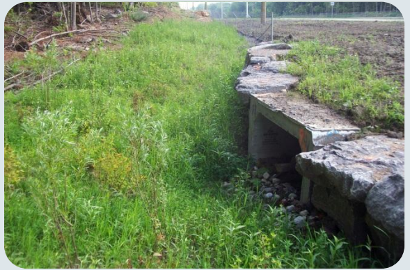
PHOTO 9: Wildlife Guide System Culvert
