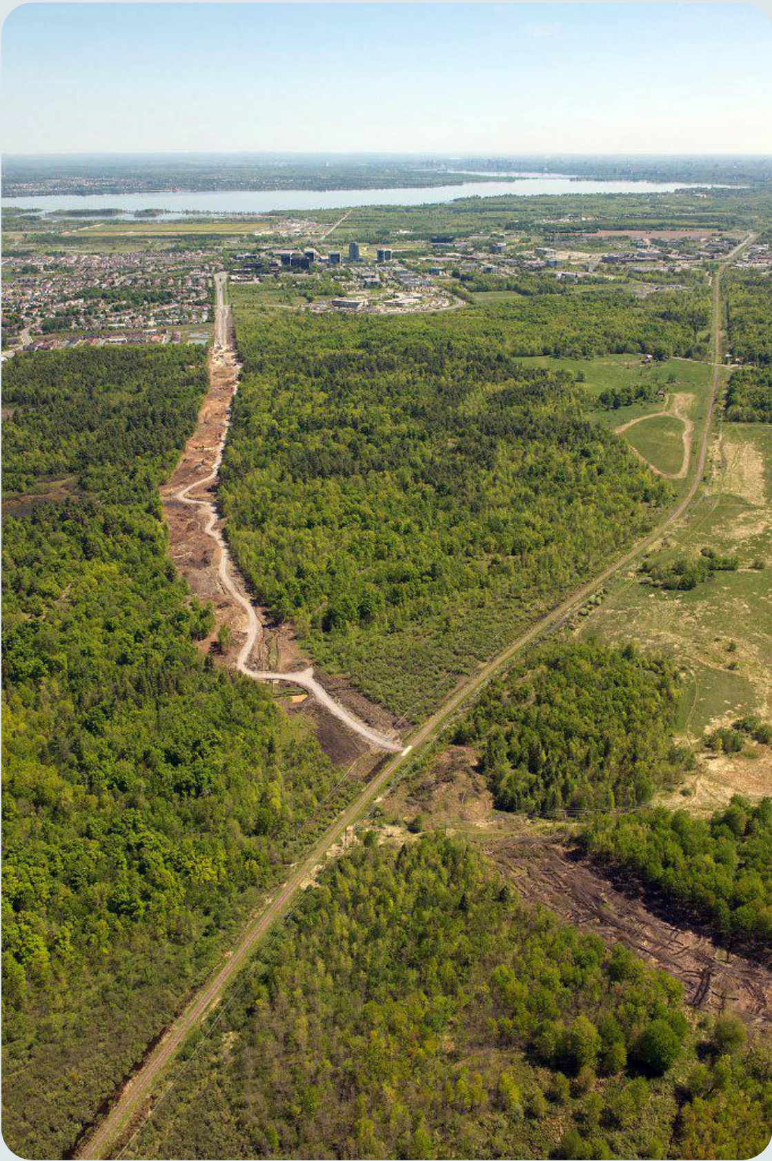
PHOTO 24: Terry Fox Drive, North east aerial view during spring construction
