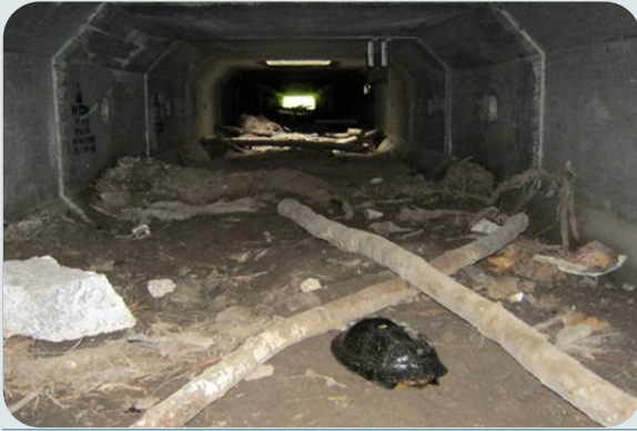
PHOTO 6: Blanding's Turtle in a Culvert
