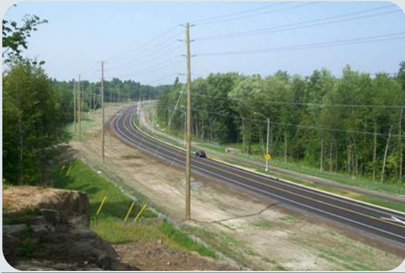
PHOTO 1: Terry Fox Drive, Completed
