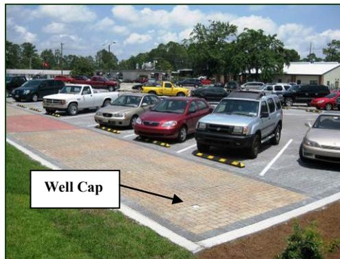
**Figure 9b. Well cap flush with the pavement surface**
