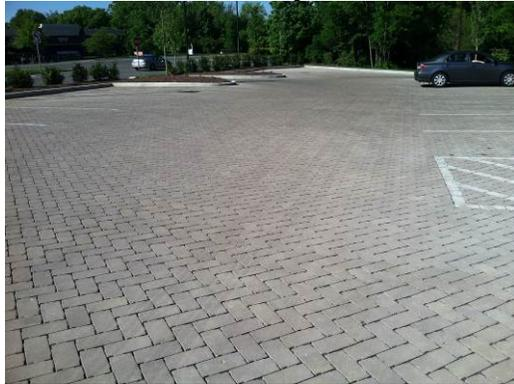
**Permeable Interlocking Concrete Pavement**
