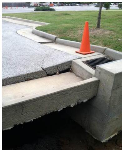
**Figure 11. Pavement failure due to water erosion of the base and subgrade**
