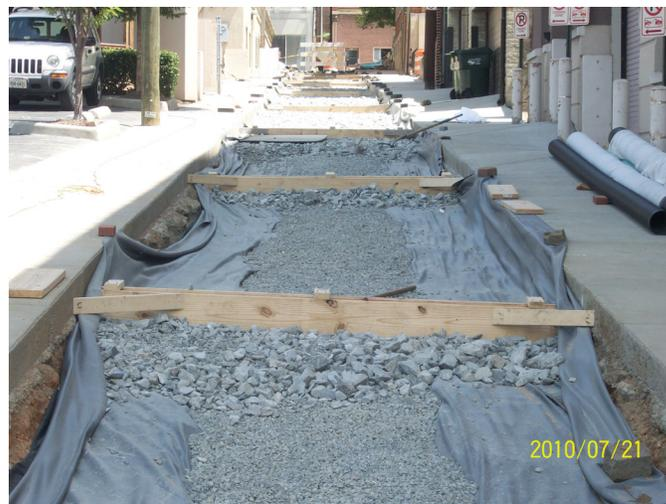
**Figure 4. Check dam construction for a permeable alleyway**
