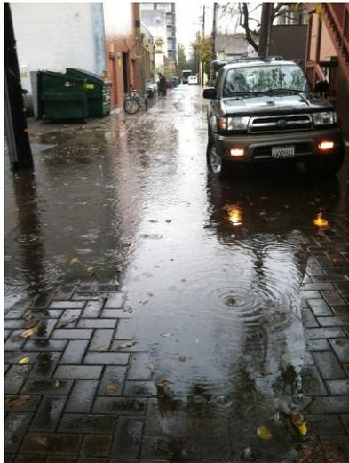
**Figure 12a. A clogged surface or an undersized drain at low-point unable to accommodate rainwater**
