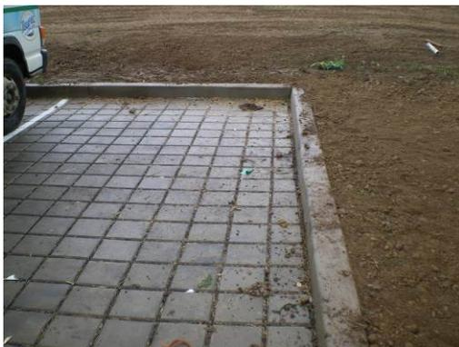
**Figure 5a. Landscaping sloping to pavement and contaminating joints**
