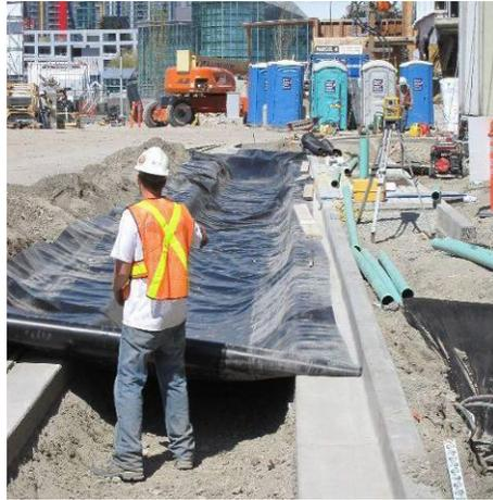
**Figure 6. Geomembrane installation**
