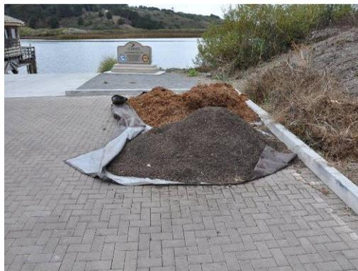
**Figure 5b. Pavement protected by placing landscaping materials on tarps**
