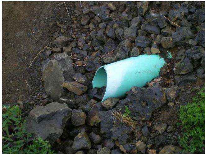
**Figure 8. Non-perforated outlet pipe surrounded by rip-rap erosion protection**
