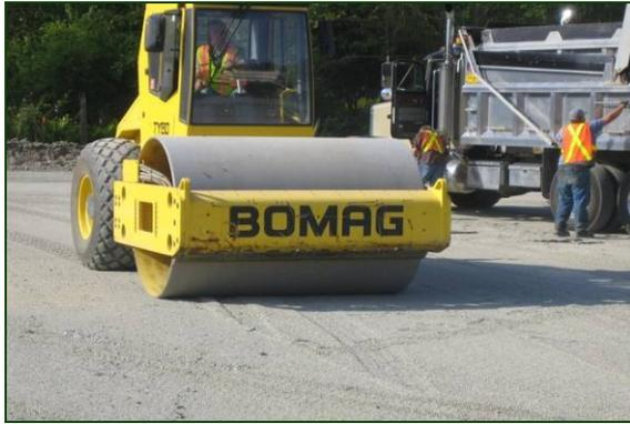
**Figure 10a. Appropriate compaction equipment for open-graded aggregate and project size**
