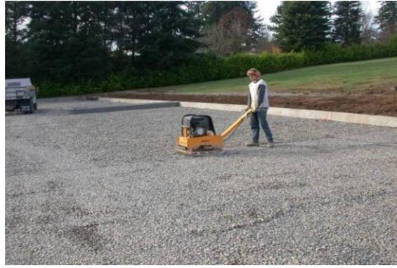
**Figure 10b. Inappropriate equipment (too small for project size) for compaction of open-graded aggregate**
