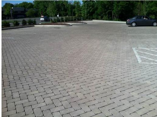
**Permeable Interlocking Concrete Pavement**
