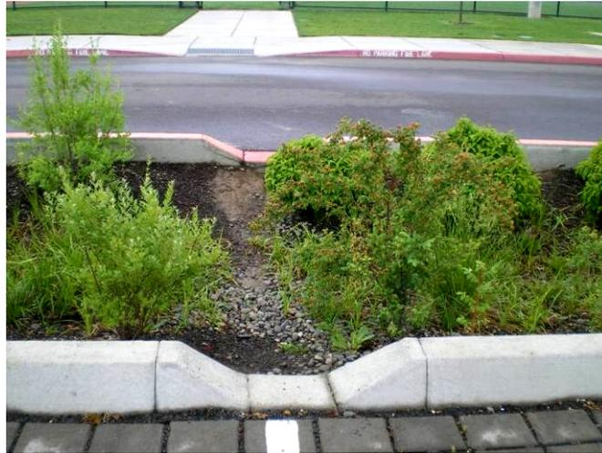
**Figure 7. Example of a curb cut-out enabling excess runoff to drain to a bioswale for additional treatment**
