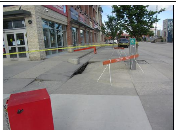
Undermined Sidewalk at 1 st St. SE and 15 Ave. intersection
