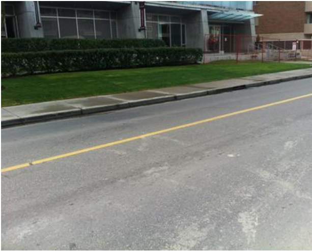
Cracked sidewalk along 25 th Ave. SE, West of 1 st St SW (Post Flooding)
