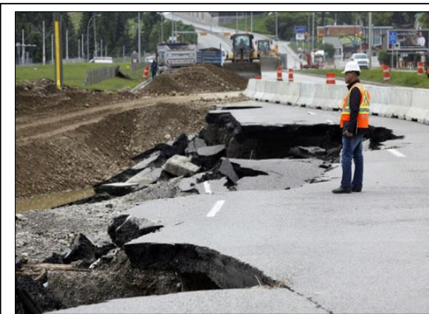
Washed out portion of Macleod Tr. at Victoria Bridge
