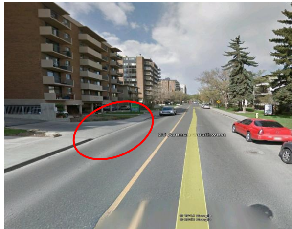
Imagery acquired from Google Earth Pro. Image dated May 2012. Distress free pavement surface.
