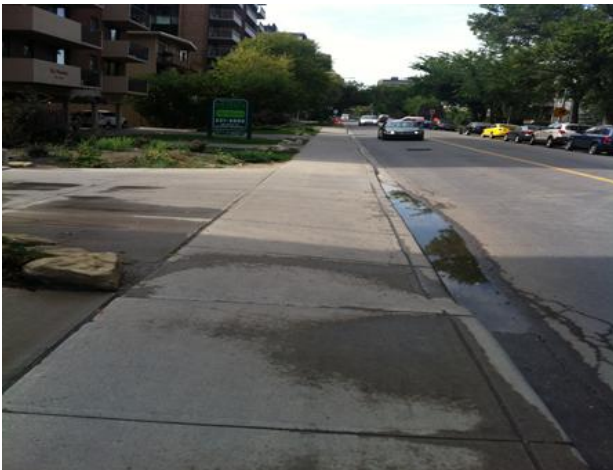
Distressed pavement along 25 th Ave S, East of 1 st St SW, South side of the road.
