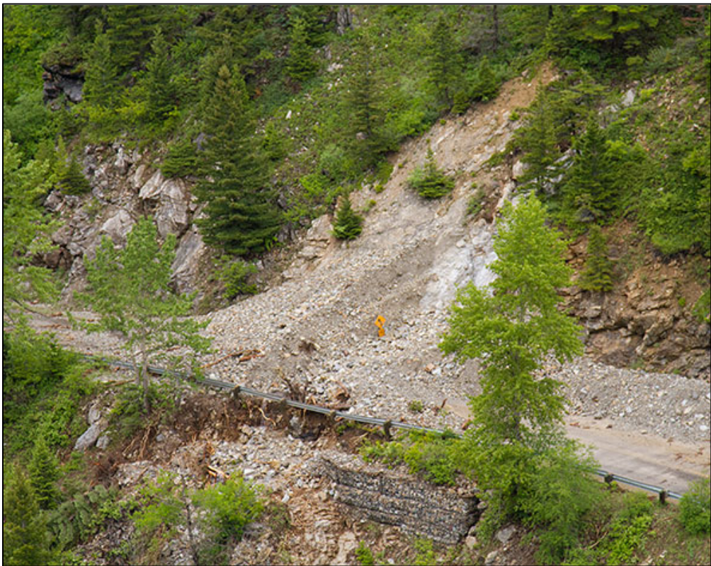
Photo 2: Debris deposited on Akamina Parkway and failure of fill slope retaining wall
