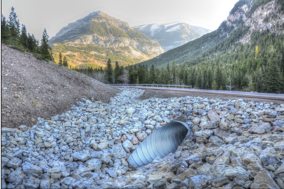
Photo 5: Inlet end of new culvert installation and associated debris storage basin
