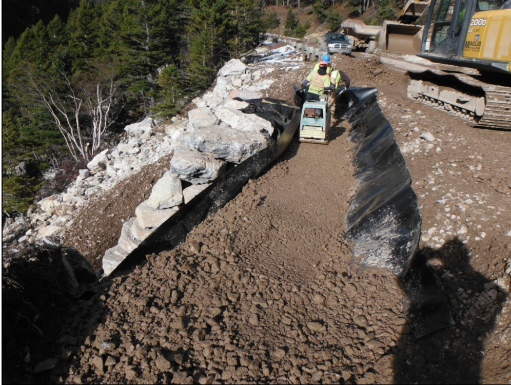
Photo 10: Construction of new fill slope retaining wall
