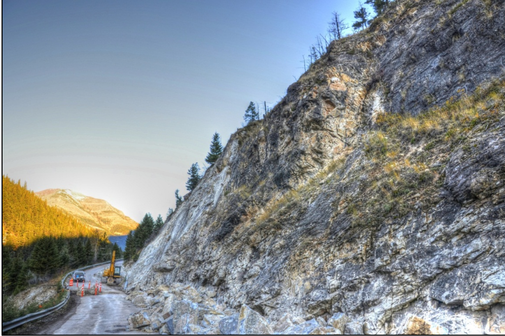
Photo 6: Rock scaling along the Akamina Parkway
