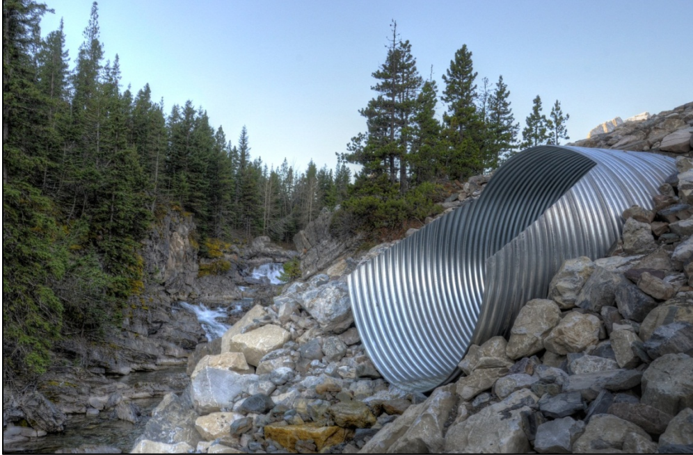
Photo 4: New culvert installation to replace effected location
