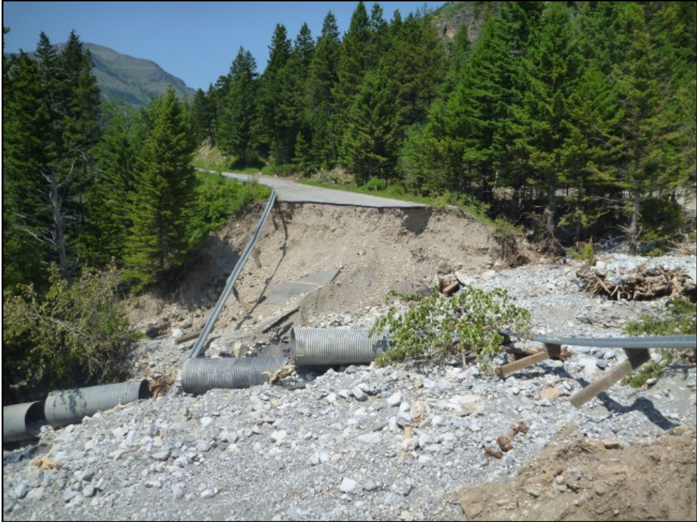
Photo 1: Typical washout of the Akamina Parkway following June 2013 Flood
