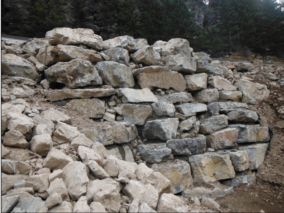
Photo 9: Newly constructed stacked boulder wall to support failed Akamina Parkway fill slope
