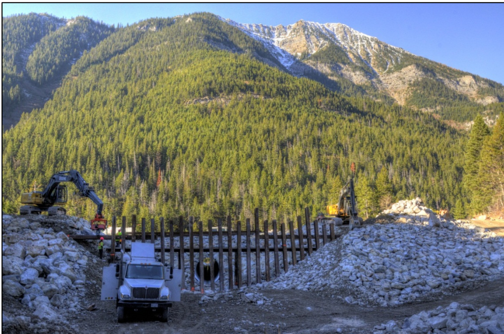
Photo 8: Installation of new trash rack and debris basin/berm
