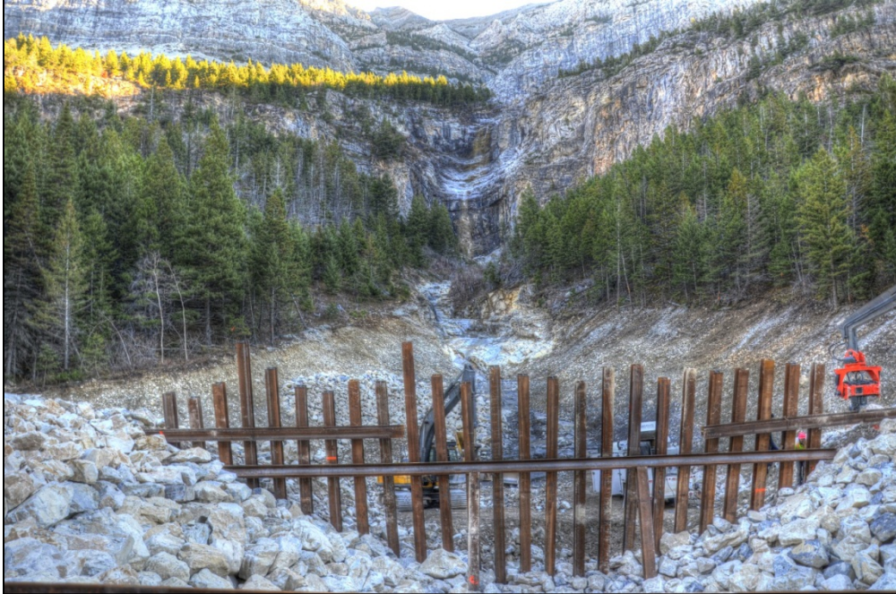
Photo 7: Newly excavated debris basin and trash rack at debris flow prone catchment
