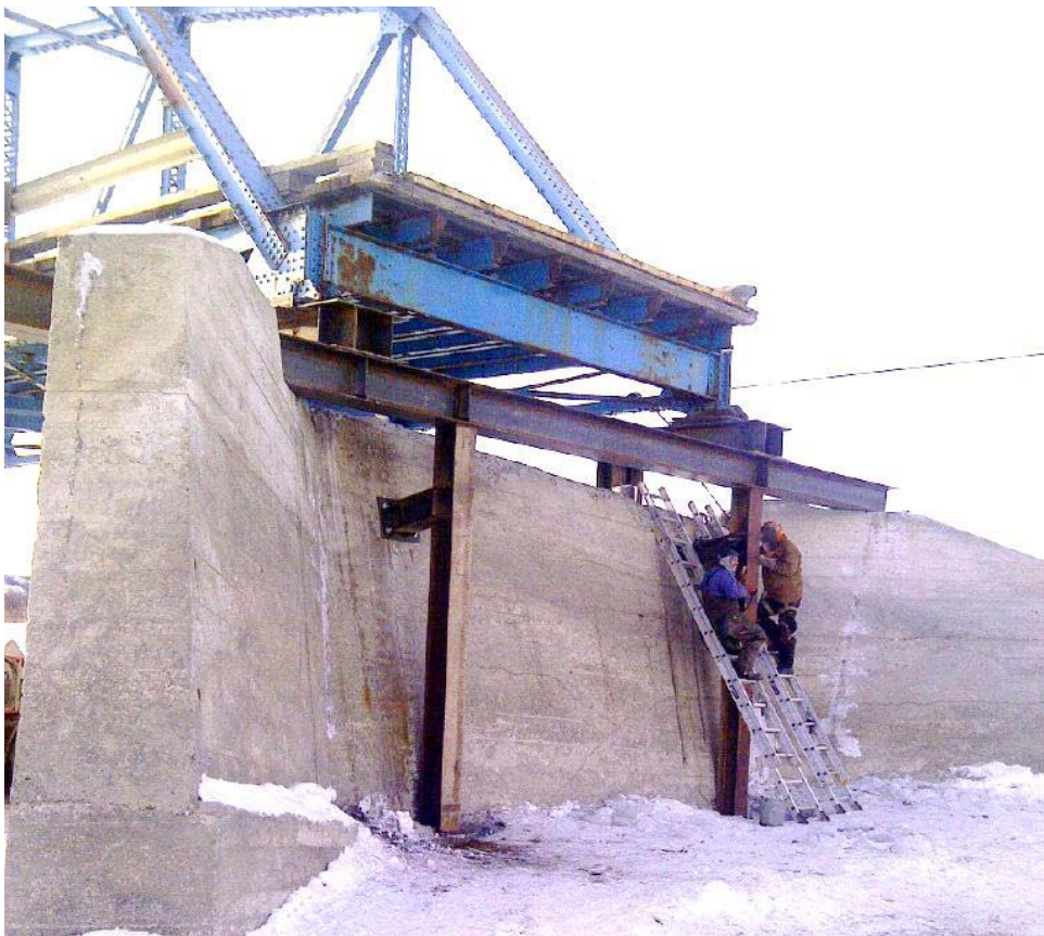
Figure 10: Stabilized on Existing Abutment
