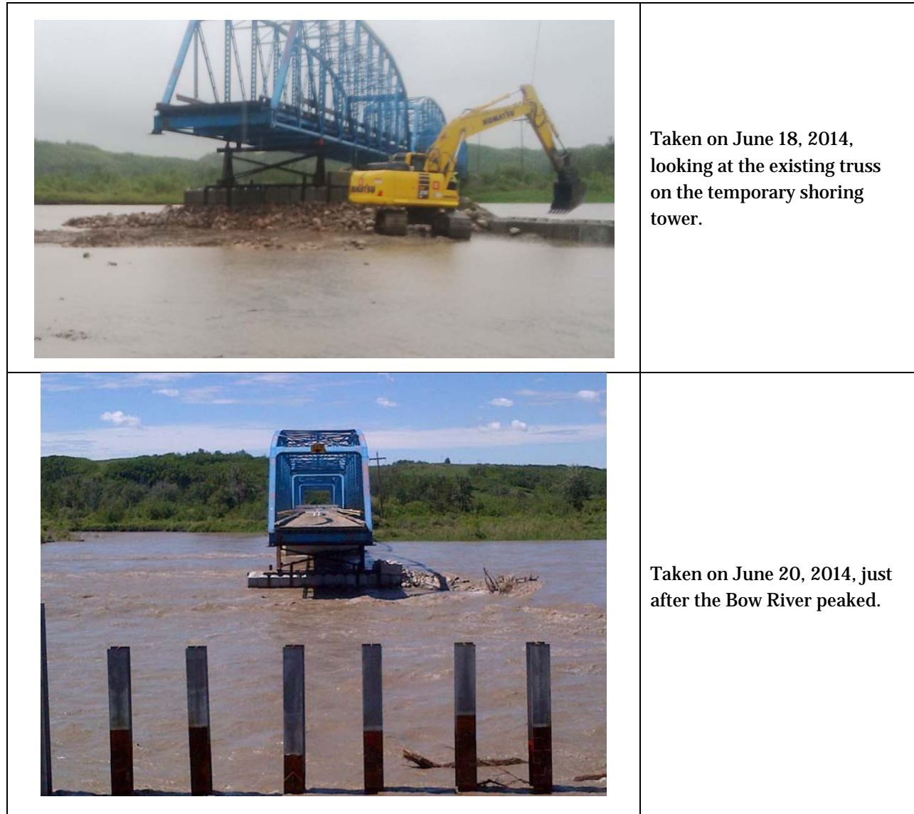
Figure 14: Shoring Tower under High Water Conditions
