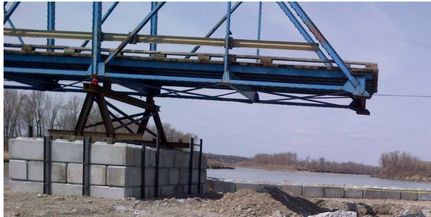
Figure 13: Shoring Tower under L2
