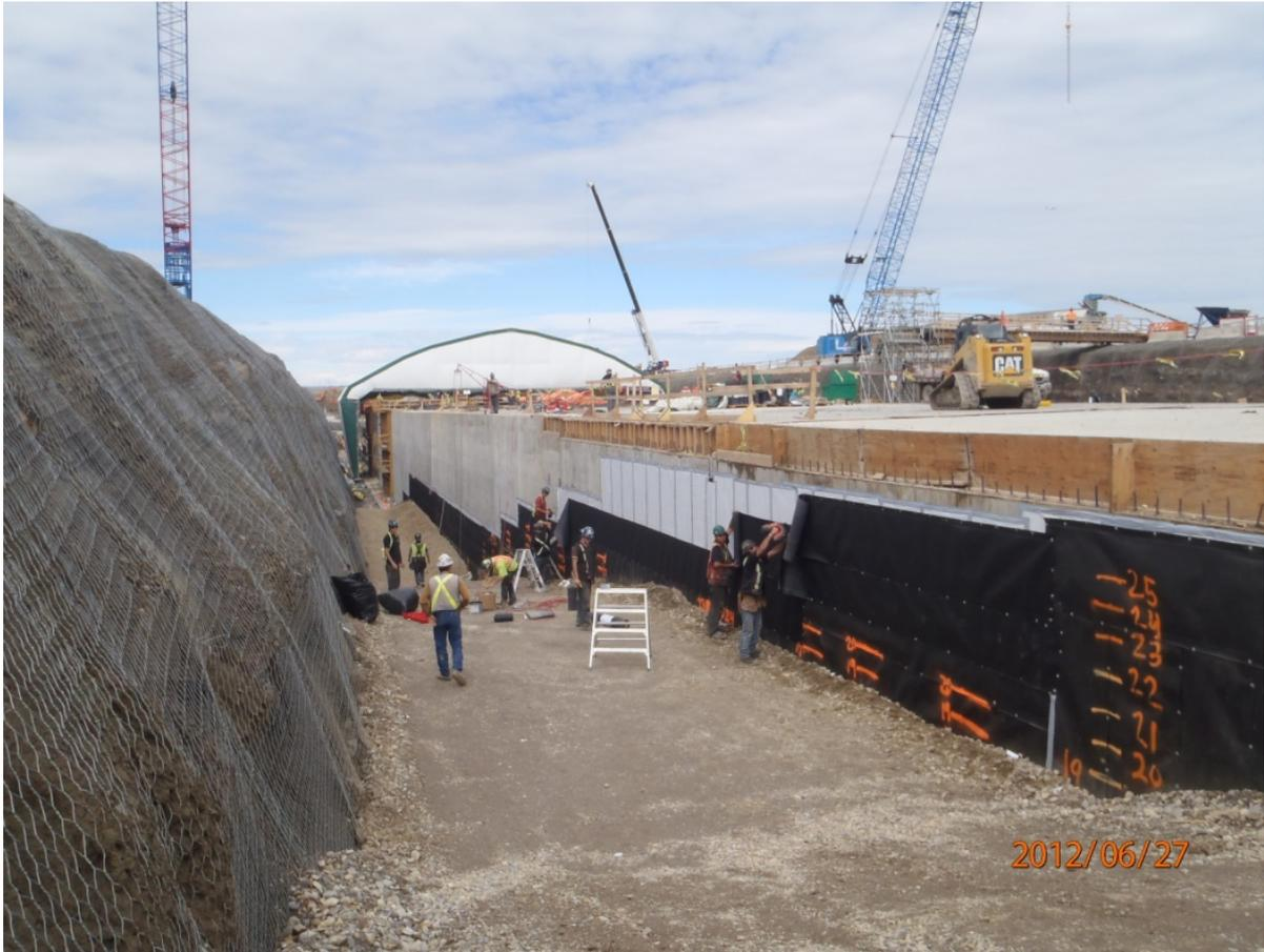
FIGURE 10 – STEPPED INSTALLATION OF TUNNEL WATERPROOFING SYSTEM AND BACKFILL
