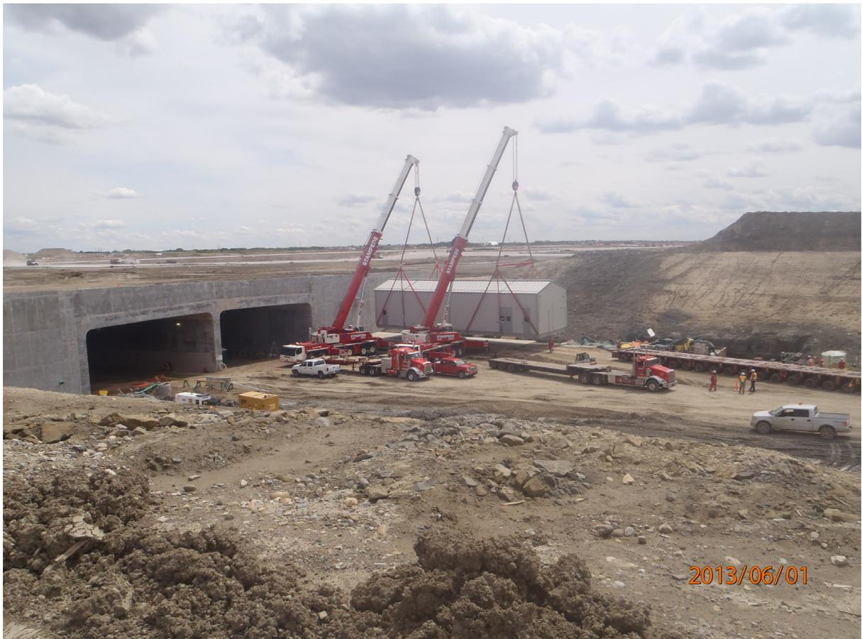
FIGURE 13 – USING CRANES TO INSTALL THE WEST CONTROL BUILDING
