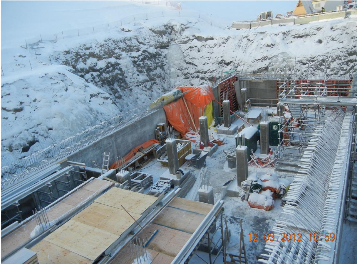
**FIGURE 8 – STORMWATER LIFT STATION UNDER CONSTRUCTION – NOTE DEPTH OF EXCAVATION**
