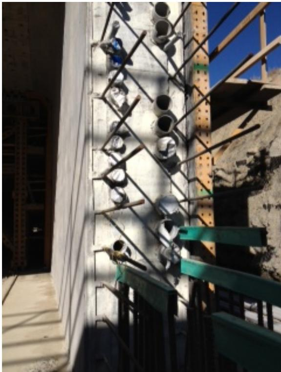
FIGURE 11 – AREA OF HIGH CONDUIT DENSITY IN TUNNEL WALL
