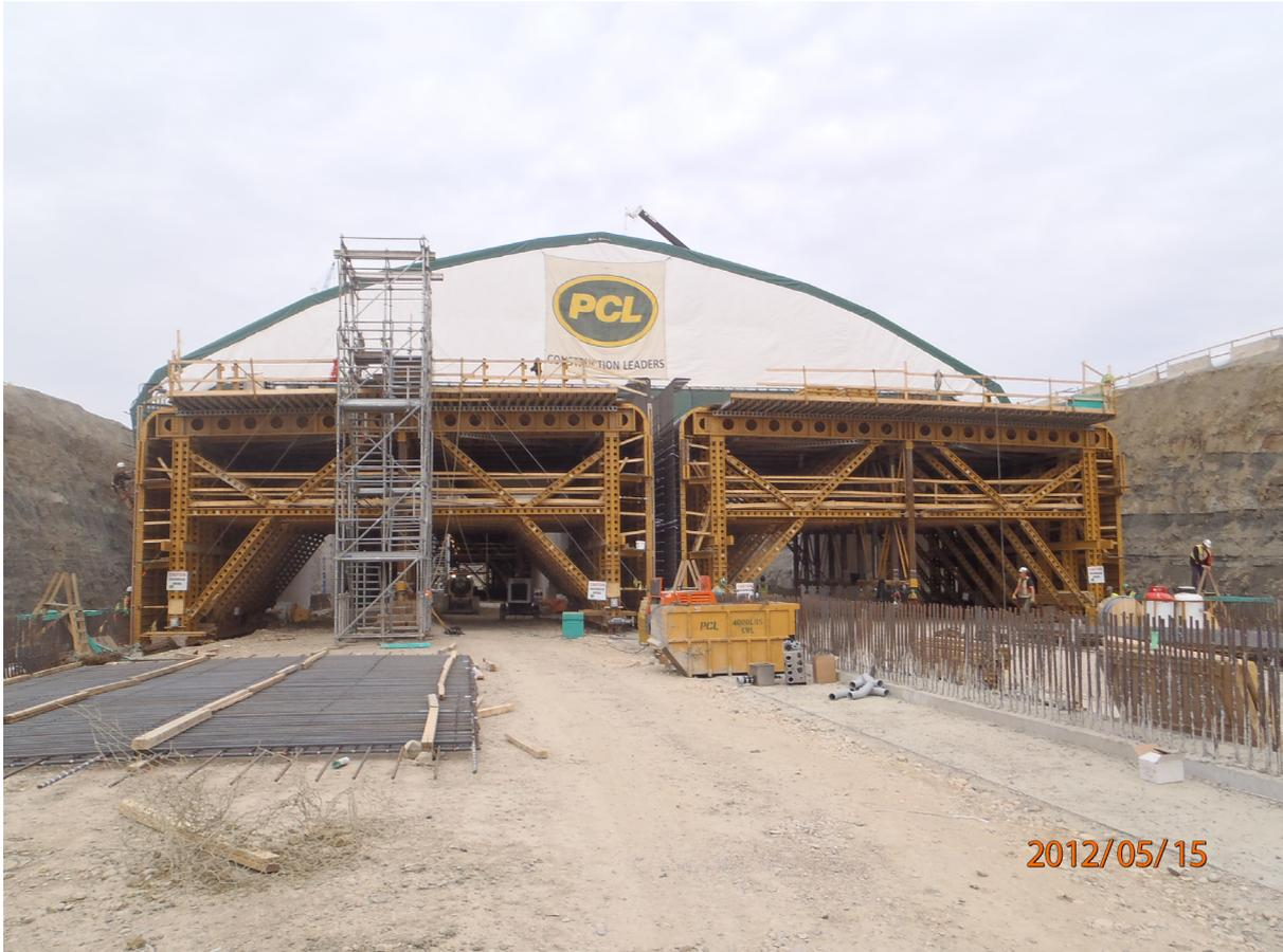
**FIGURE 6 – STEEL FORMWORK AND HORDING TENT USED FOR TUNNEL CONCRETE CASTING**
