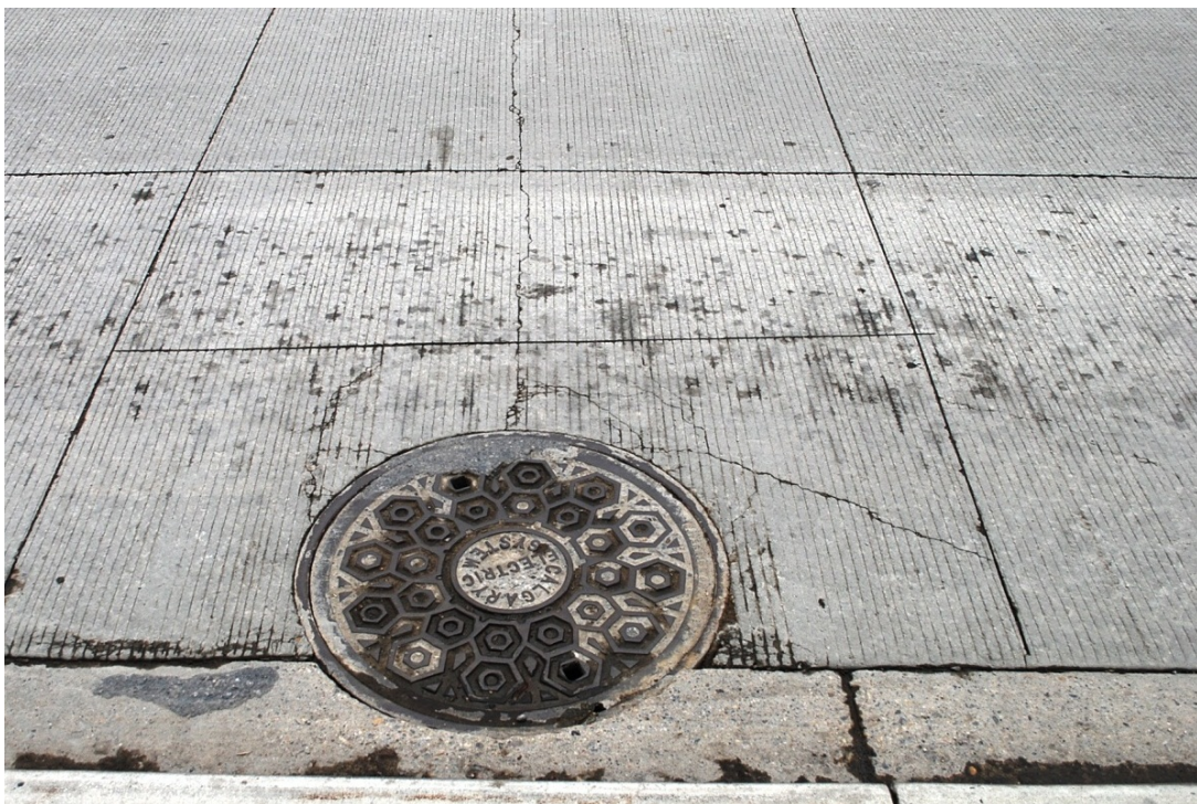
Photo 6. Transverse and random cracking around manhole
