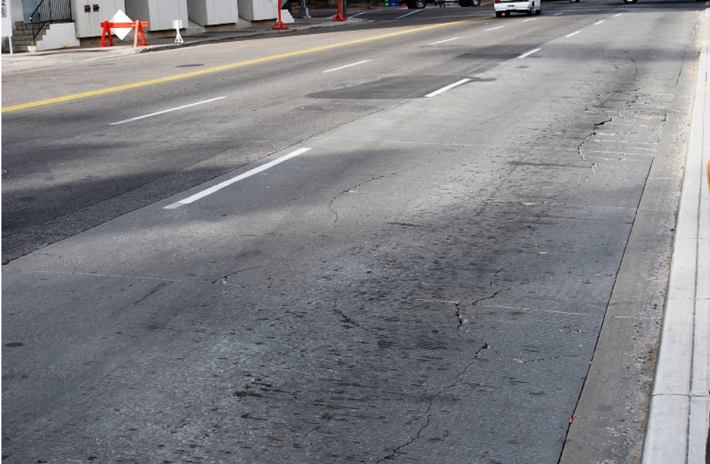
Photo 3. Cracking between tooled joints
