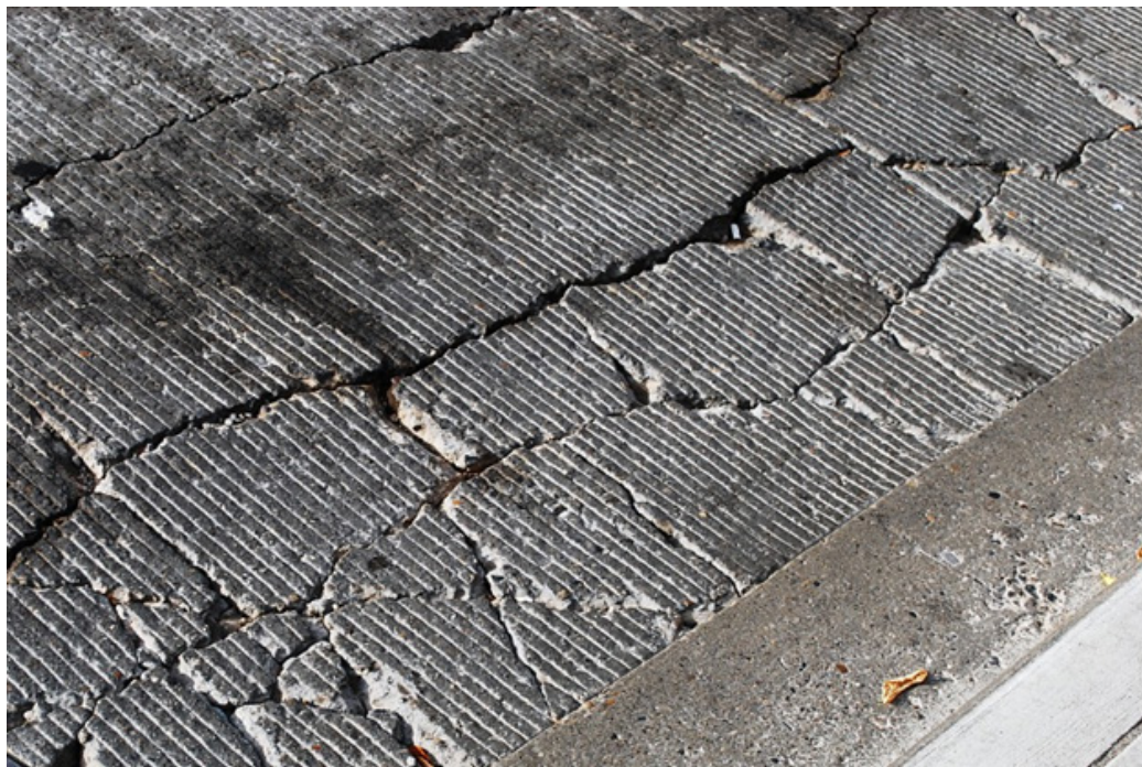
Photo 2. Concrete cracking at the bus stop
