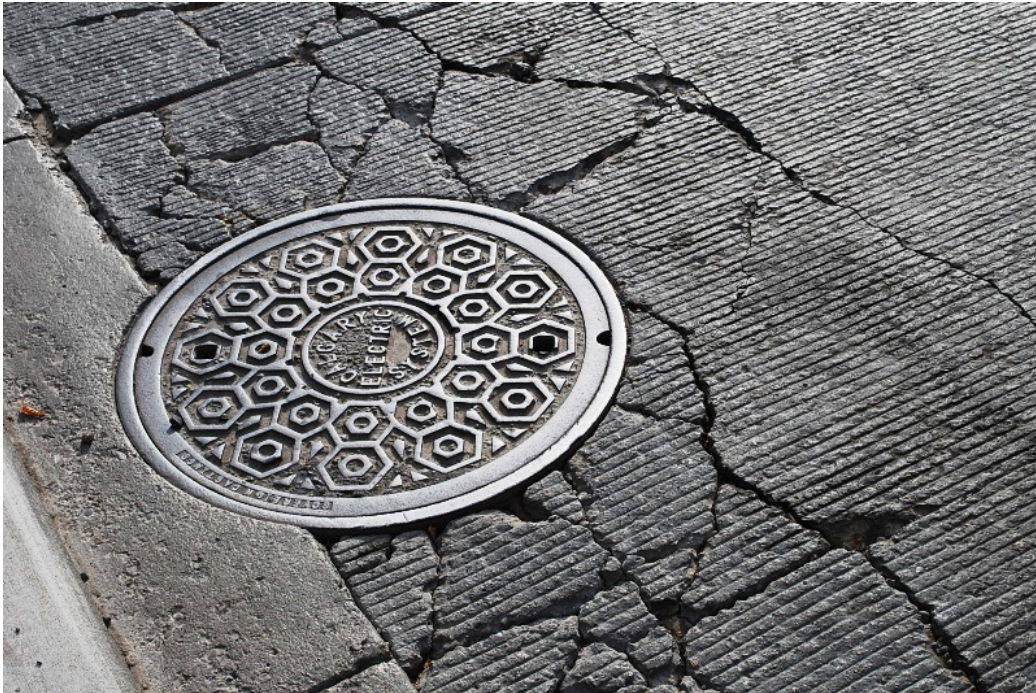
Photo 1. Extensive cracking around the manhole
