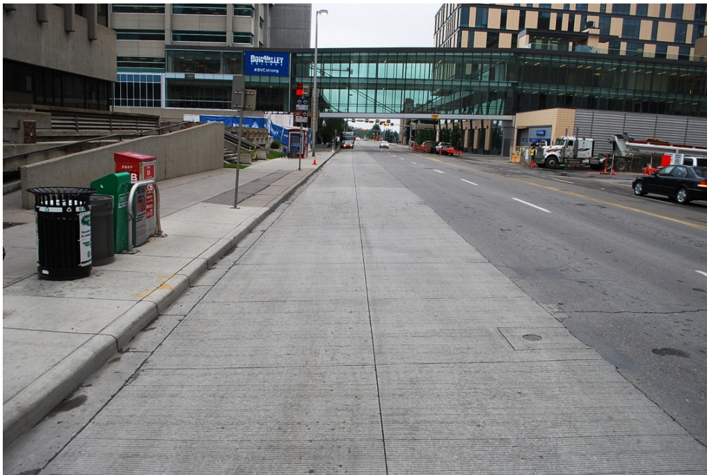
Photo 4. Concrete overlay – general view
