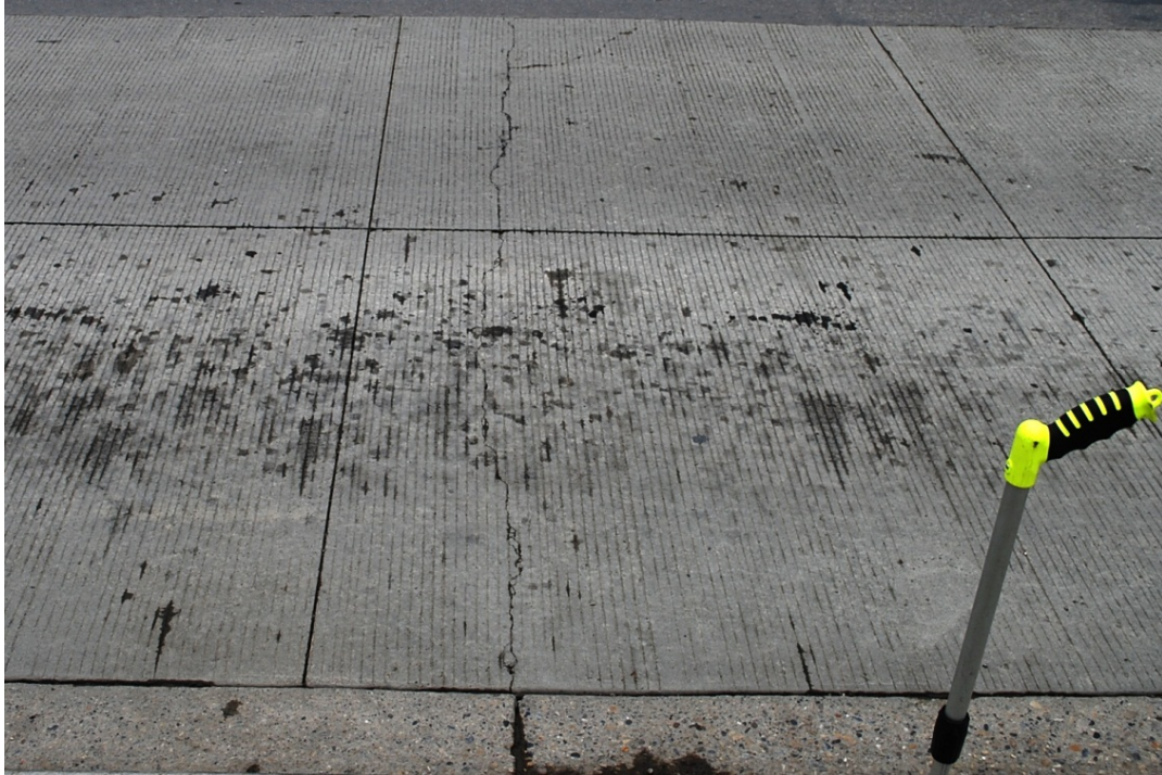
Photo 5. Preferential crack at adjacent sidewalk control joint
