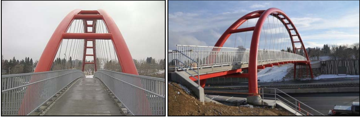
Figure 1: View of bridge deck from south abutment (left) and view of bridge from the north abutment (right).
