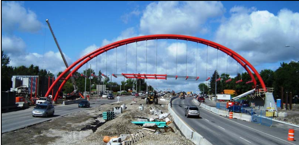
Figure 11: View of bridge, following arch erection, prior to erection of precast deck panels and placement of cast-in-place concrete topping.
