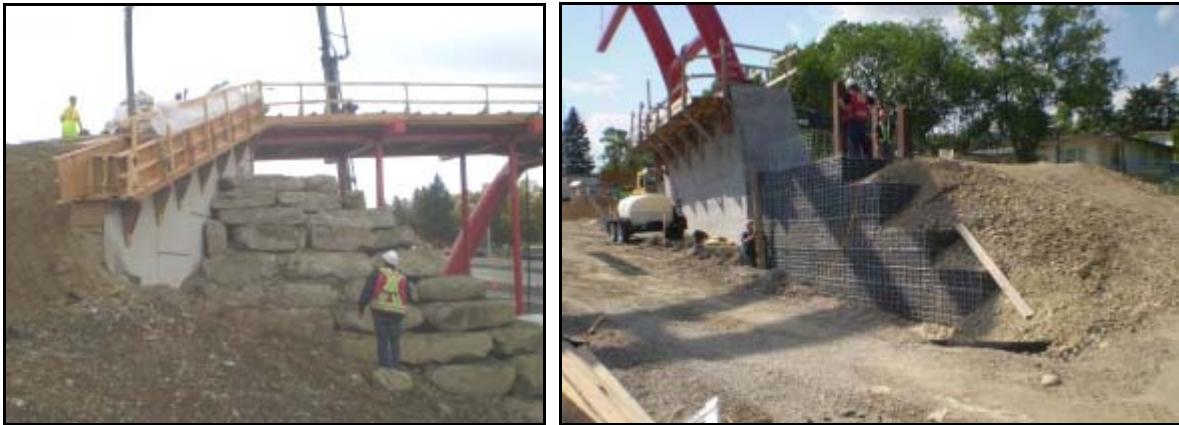
Figure 7: View of the south abutment, utilizing a rock-stack wall for improved slope appearance (left) and the north arch foundation and adjacent 2-stage MSE wall facing (right).
