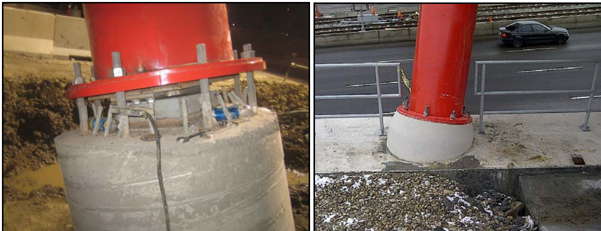
Figure 12: View of temporary bearings just after arch erection (left) and following grouting to achieve fixity (right).
