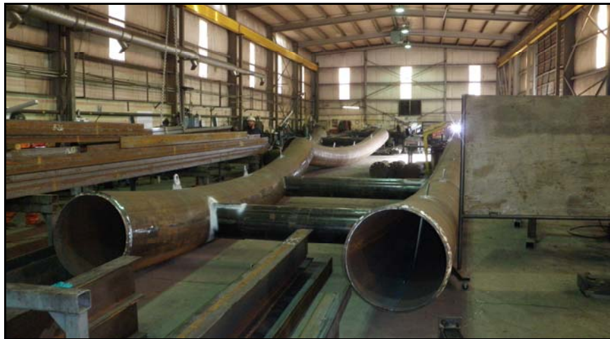
Figure 8: View of fabrication of the arch sections in the shop.
