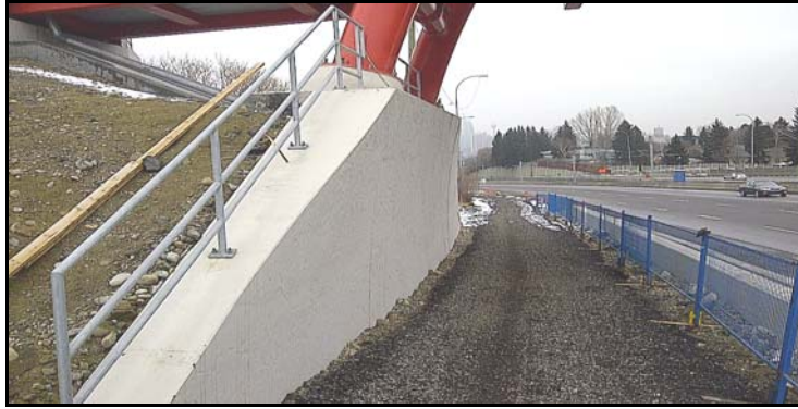
Figure 13: View of North arch foundation and curved retaining walls.
