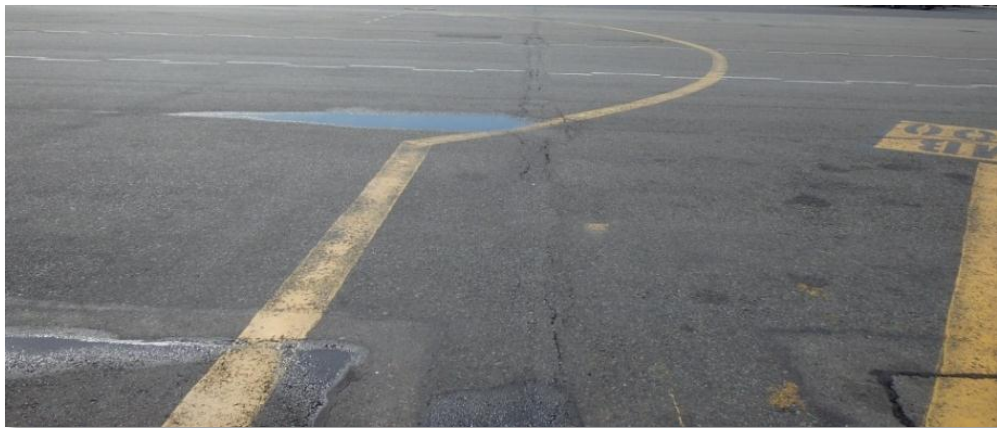
Figure 3: Low Severity Fatigue Cracking
