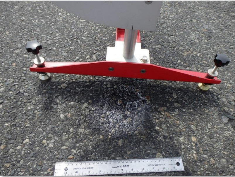
Figure 6: Unsealed Asphalt Pavement
