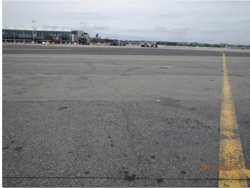
Figure 4: Low Severity Linear Crack
