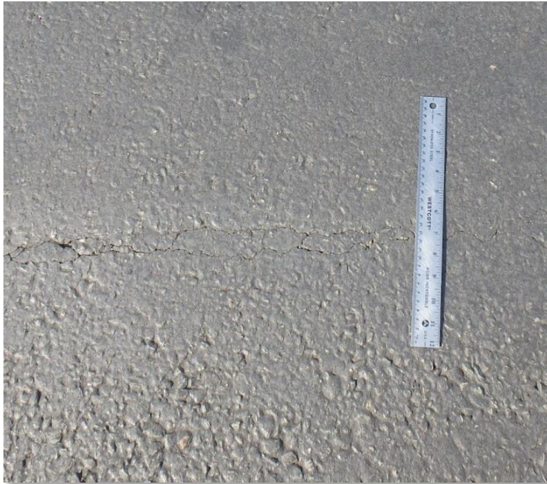
Figure 1: Low Severity Linear Crack and Asphalt Sealant
