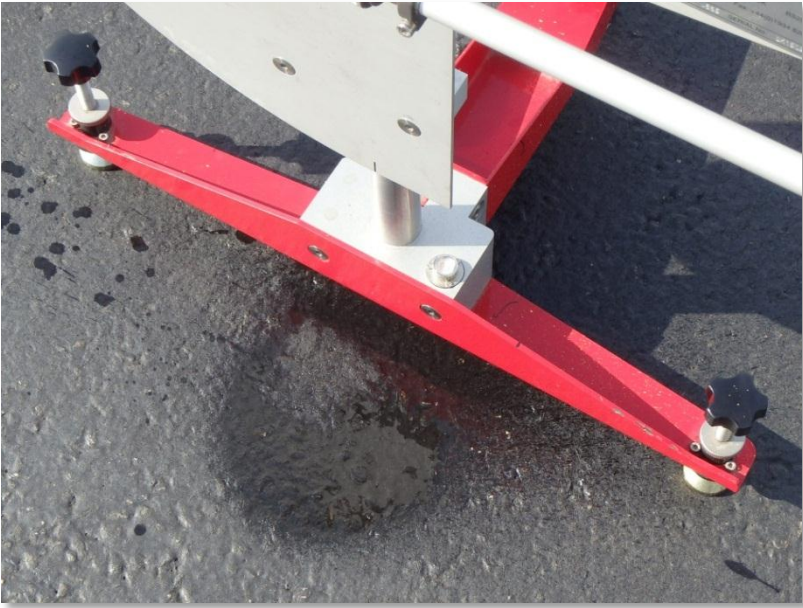
Figure 7: Sealed Asphalt Pavement
