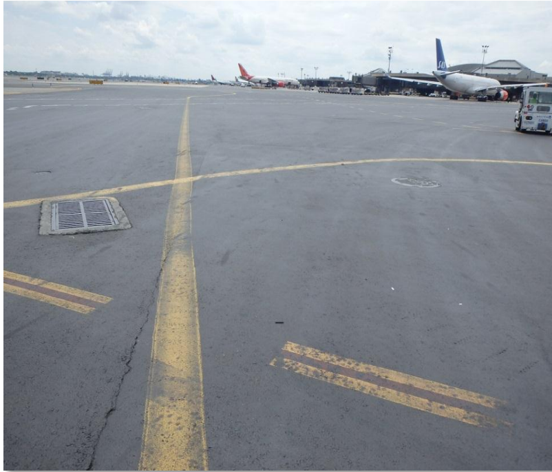
Figure 2: Low Severity Linear Crack
