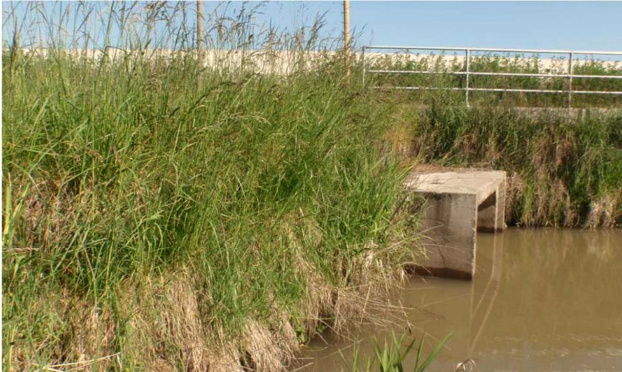
Photo H: RSS wing wall at box culvert 3 years post construction [May 2015]
