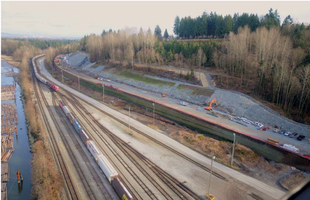
Photo H: 8M HIGH RSS SLOPE, LOOKING EAST ALONG THE FORESHORE OF THE FRASER RIVER
