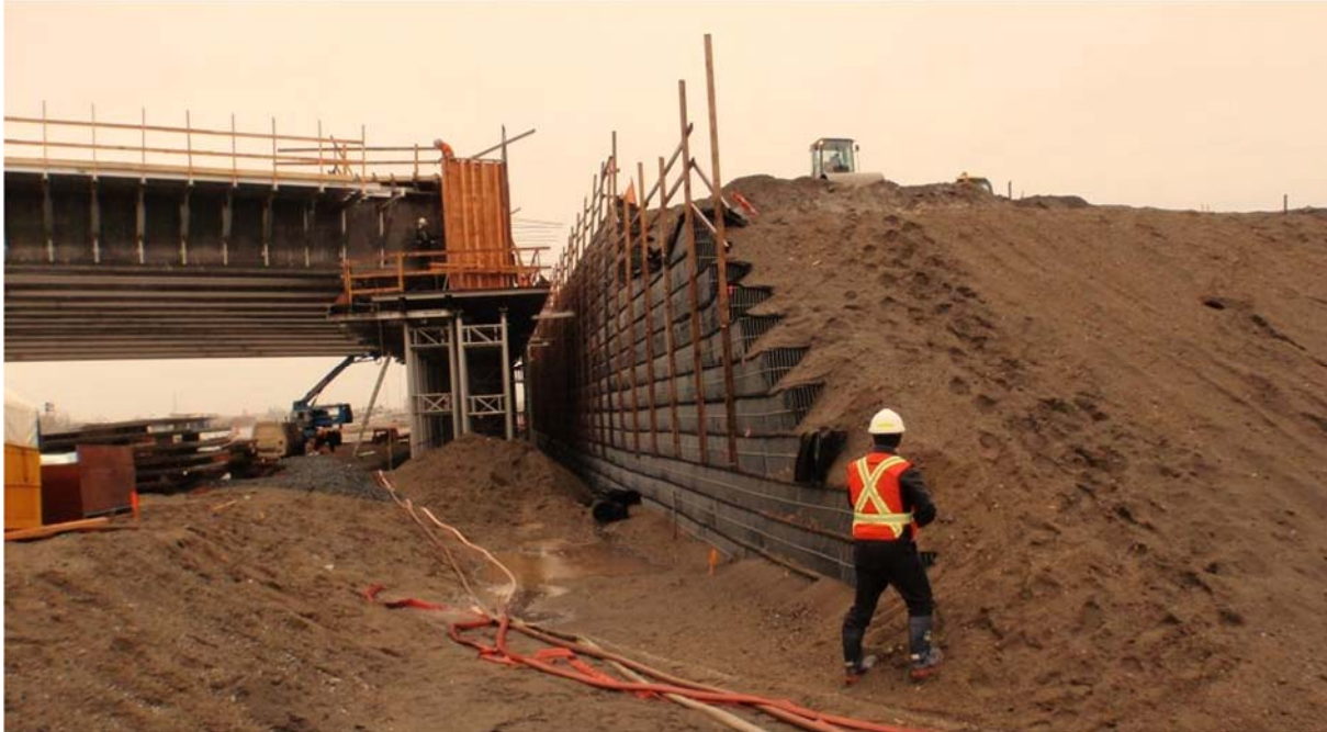
Photo C: North Abutment at Structure 8225, 1 st Stage Wire Wall Earthworks Proceeding, February 2013
