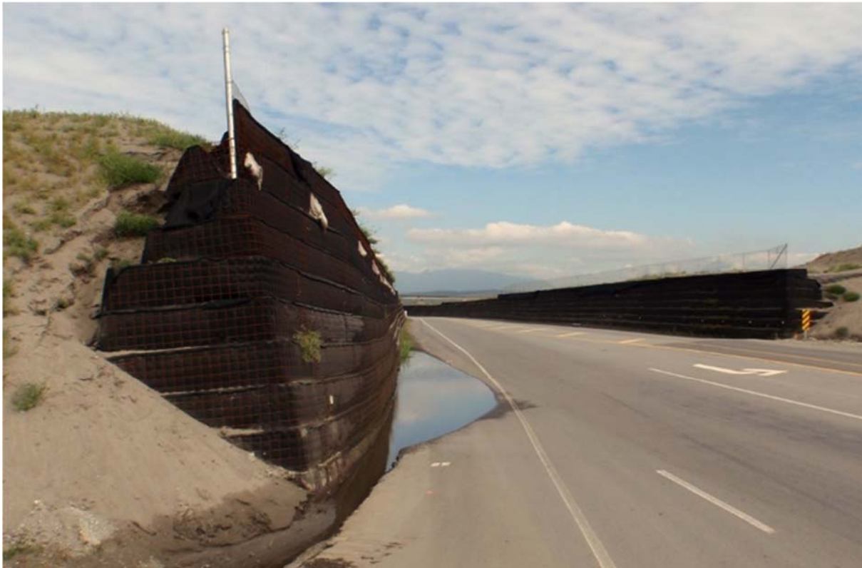
Photo A: Preload Walls Comprised of Welded Wire Facing, Geotextile, and HDPE Soil Reinforcement
