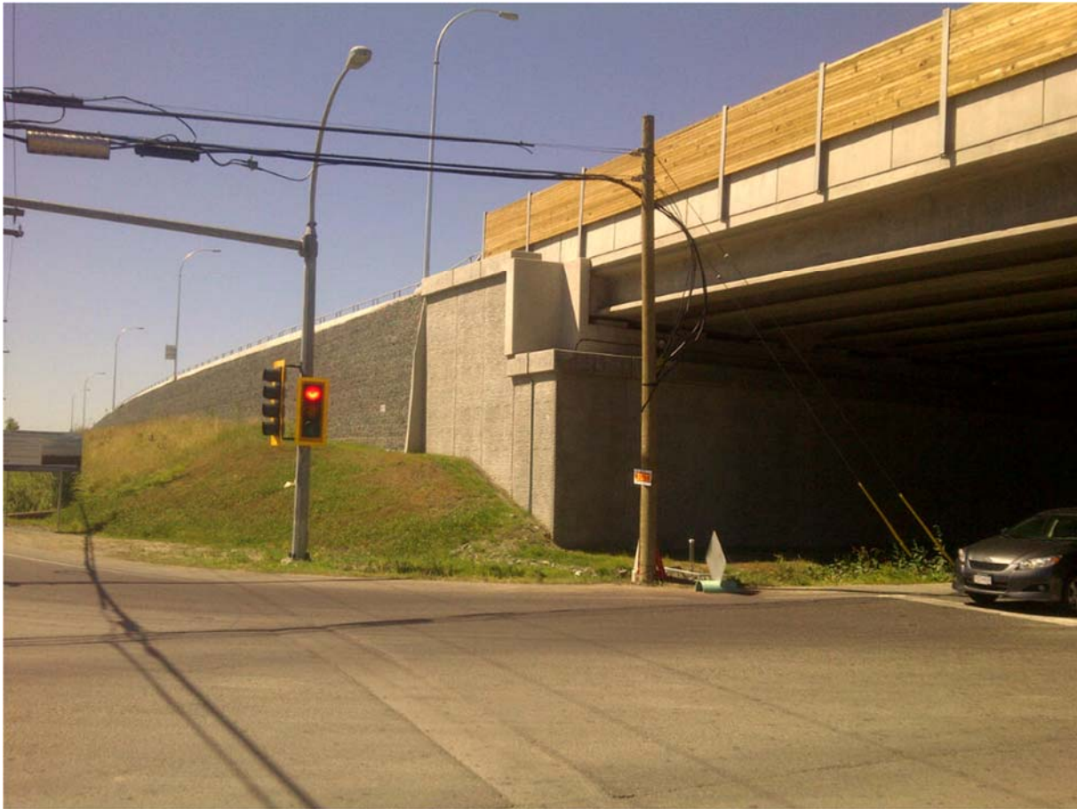
Photo B: SierraScape® Galvanized Wire-Faced Walls (Left Hand Side) Leading Up To MSE Bridge Structure
