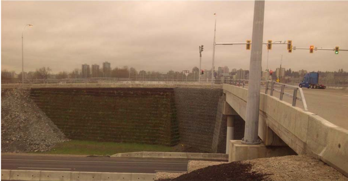
Photo I: Column Supported Bridge Deck with Galvanized Wire Faced Walls, and RSS Approach Slopes
