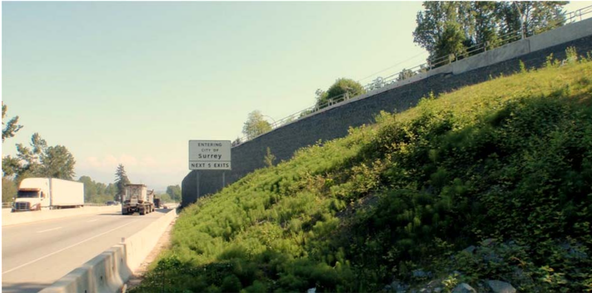
Photo courtesy of Nilex Inc. Photo G: Retaining Wall No. 8287 at Gunderson, and just above SFPR alignment [May 2015].
