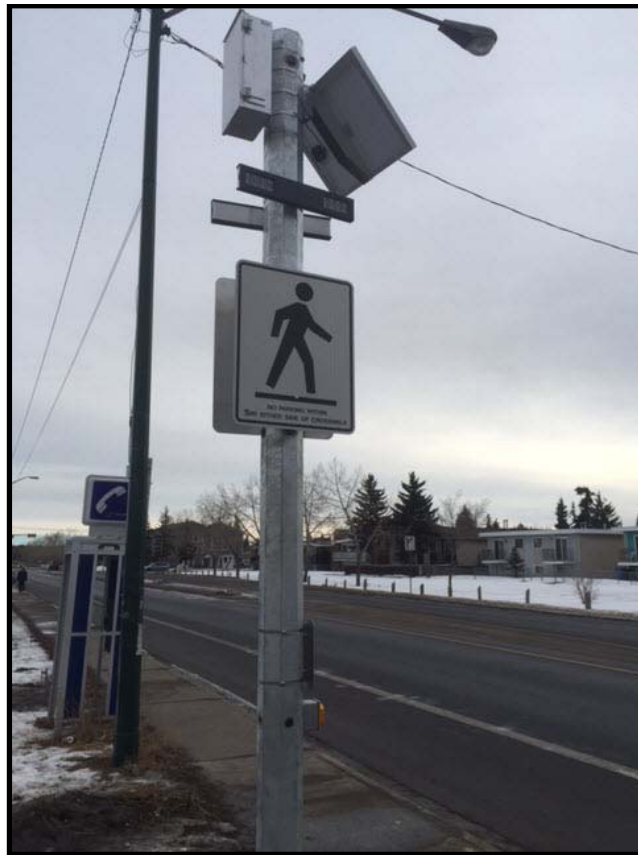
Figure 7: Phase 2 RRFB installation at Bowness RD NW
