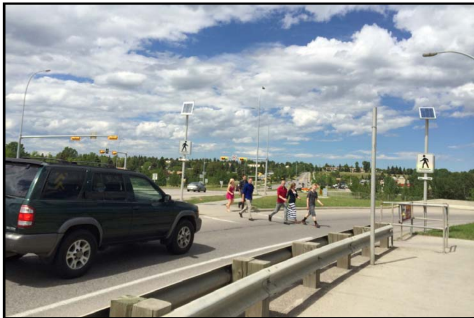
Figure 2: RRFB installed at 18 St/Glenmore Tr ramp
