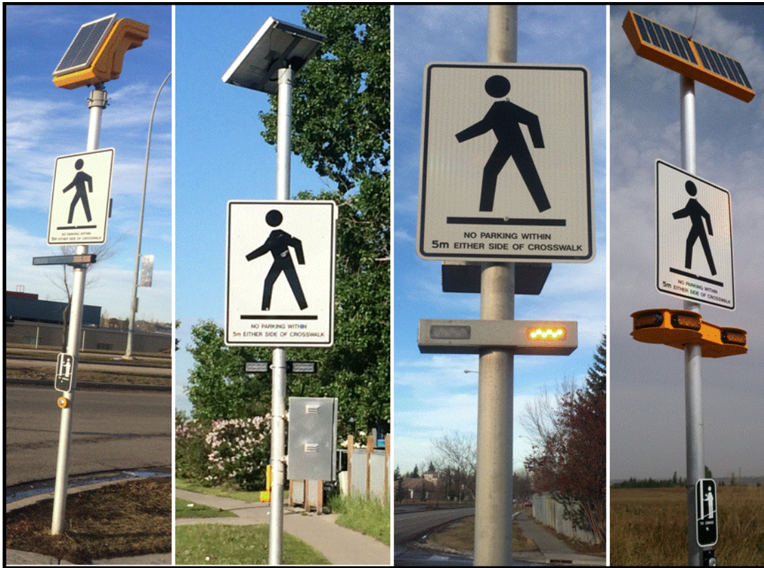
Figure 4: Various types of RRFB devices used in Calgary as part of Phase 1 Pilot
