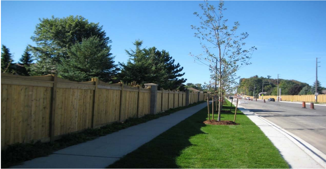
Figure 12: Shellard Lane post construction, concrete sidewalk with boulevard, wood acoustic fence and new trees
