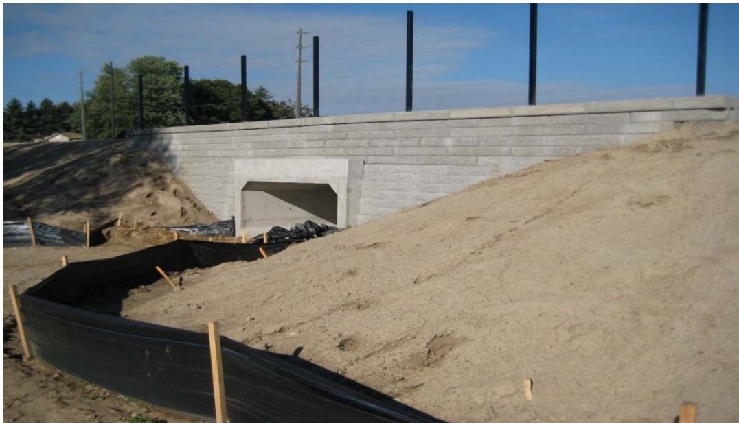
Figure 14: South headwall at Culvert 2
