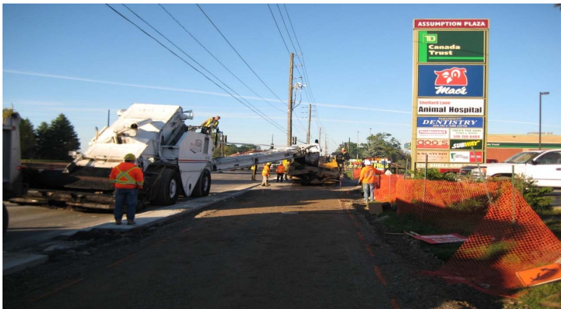
Figure 15: Paving the multi-use trail at Assumption Plaza (School Block)
