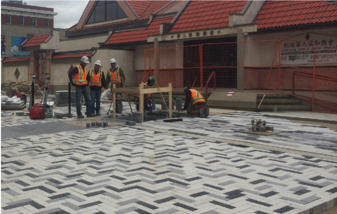
Figure 4 Flush Curb on West Side of 96 Street
