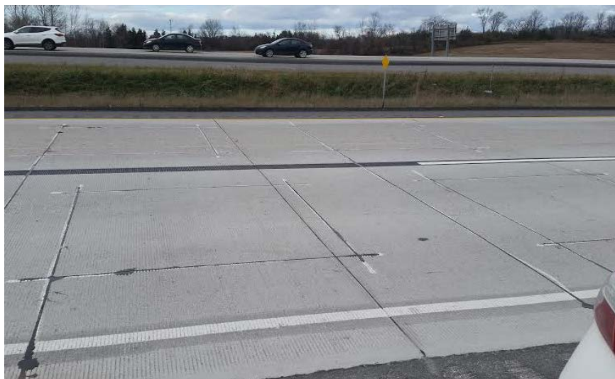
Picture 2 – Intrusive Loops on MTO's Highways
