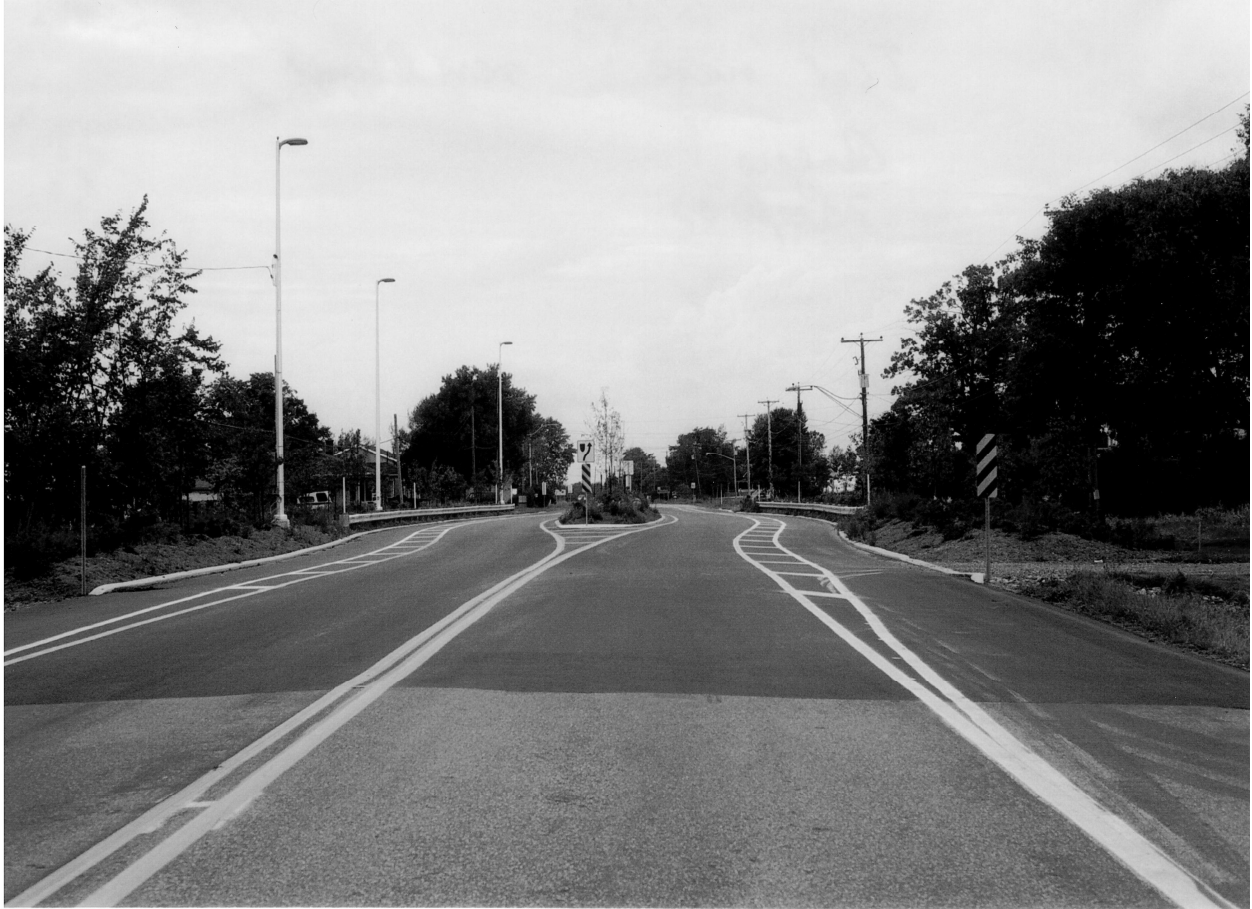
Figure 1. Speed reduction island at the western entrance to Angers
