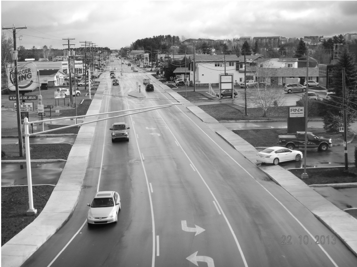
Figure 5. Two-way left turn lane and protected left-turn bays on 3 rd Avenue West in Val-d'Or (looking east)
