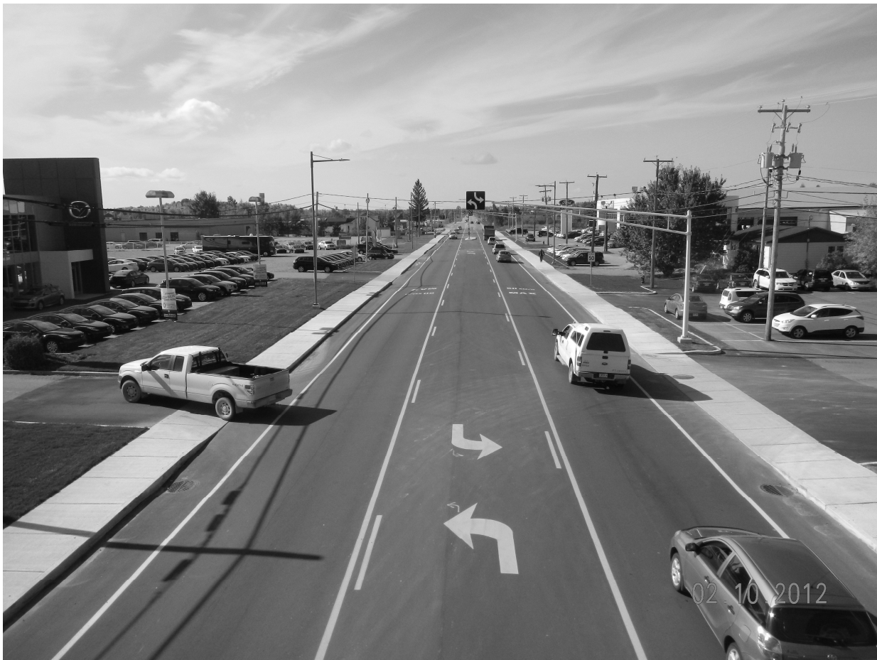
Figure 3. Two-way left turn lane on 3 rd Avenue West at the western entrance to Val-d'Or, QC (looking west)
