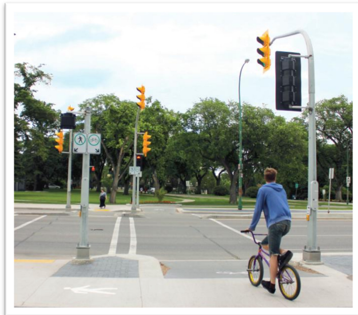
Figure 1 – Separate pedestrian and cycling signalized crossing in Winnipeg
