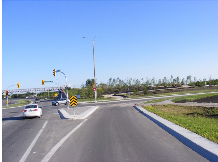
Figure 2 – Example of a smart channel in Winnipeg from an expressway to an arterial
