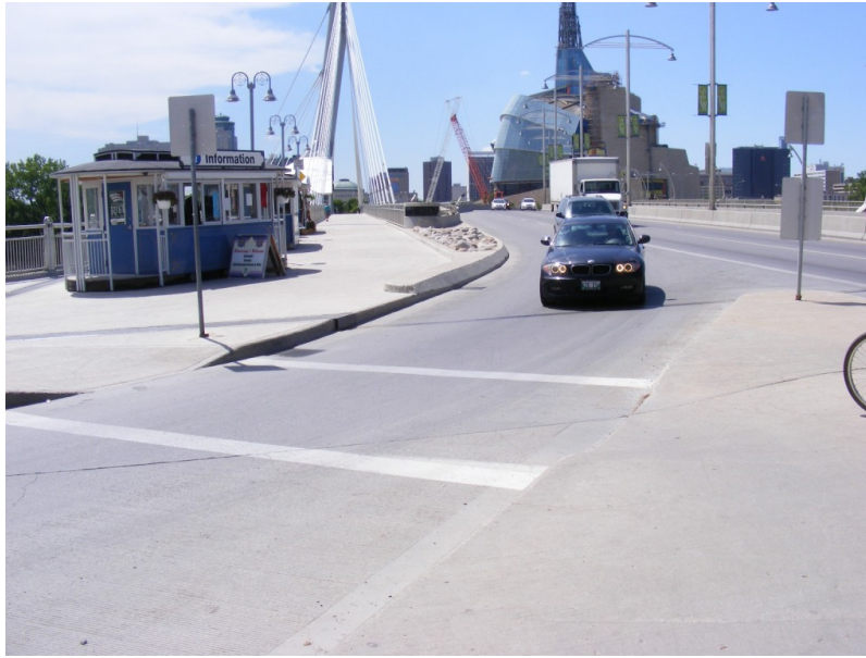
Figure 4 – Provencher Boulevard right turn onto Tache Avenue demonstrates how the downstream crossing allows for good sight lines for the driver.
