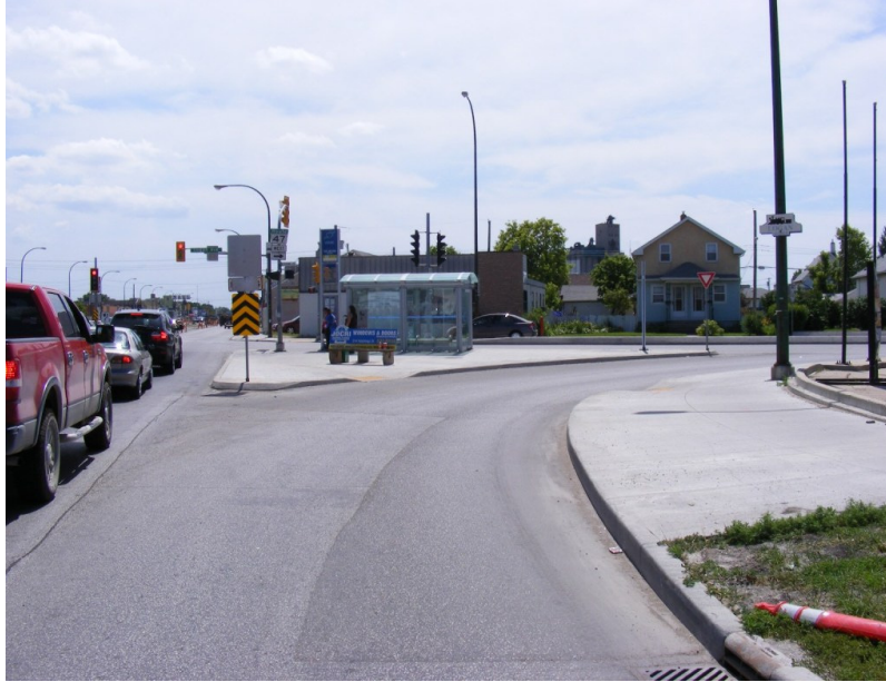
Figure 5 – McPhillips Street right turn onto Logan Avenue demonstrates the benefits of placing the pedestrian crossing upstream for visibility
