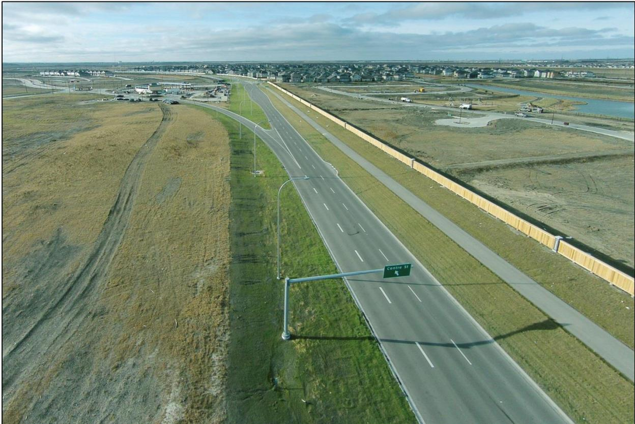
*Figure 9: OHSS moved out of clear zone to avoid need for roadside protection (guardrail).*
