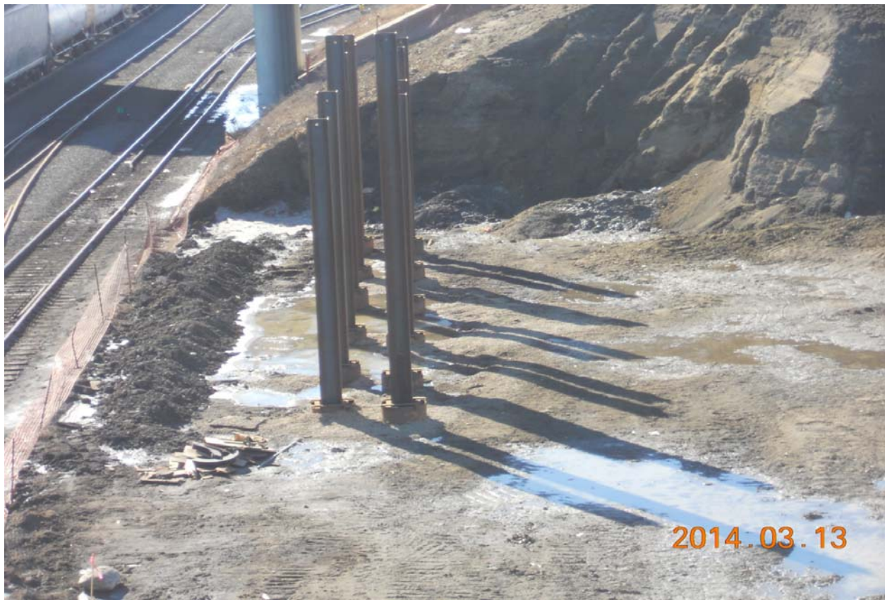
Figure 10 Successfully Installed Abutment Piles
