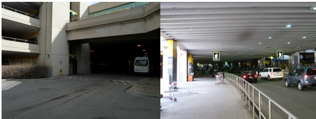
Figure 5.5 – Dark Area near Rental Car Centre (Bus Facility left, Roadway right)
