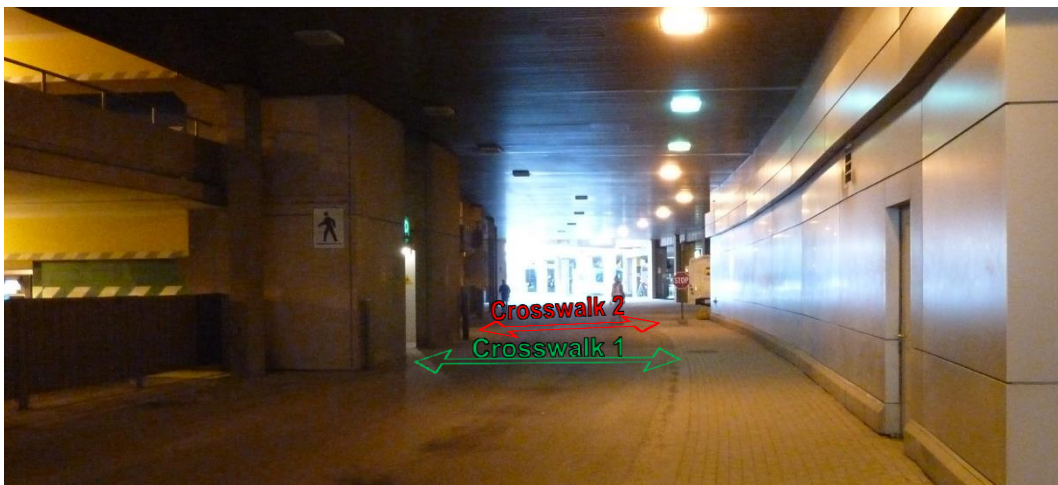
Figure 5.9– Example Poor Crosswalk Placement
