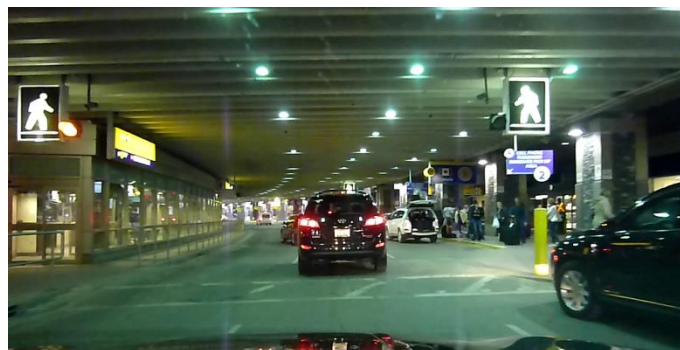
Figure 5.8 – Crosswalk with Flashing Warning Signal
