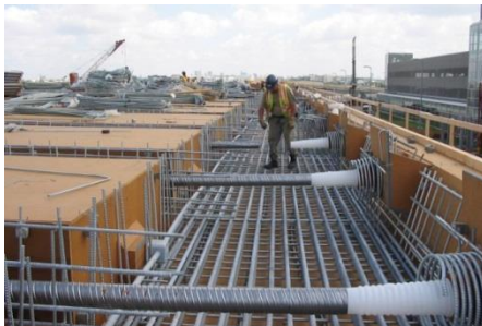
Photos 10 to 12: Post-Tensioned Transverse Beams and Thickened Edge Beam to Meet Vertical Clearance Requirements, Improve Bridge Aesthetics, and Provide Open Column Spacing
