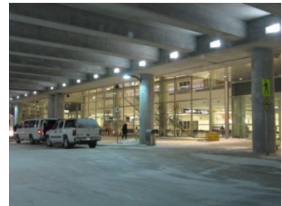
Photos 10 to 12: Post-Tensioned Transverse Beams and Thickened Edge Beam to Meet Vertical Clearance Requirements, Improve Bridge Aesthetics, and Provide Open Column Spacing
