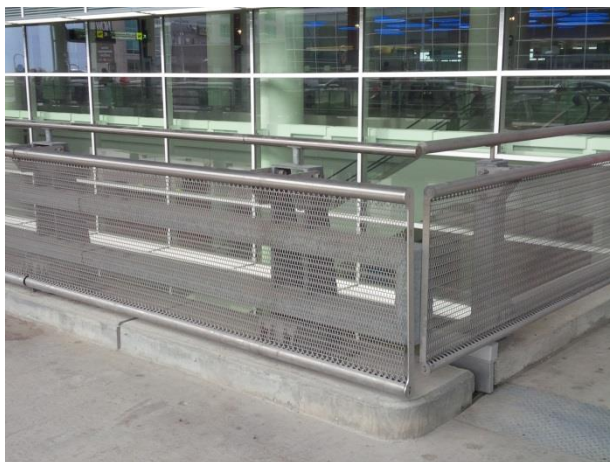
Photo 16 and Figure 7: Barrier / Railing Detail along Departures Level Sidewalk
