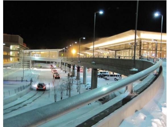
Photo 15: Aluminum Railing on Concrete Traffic Barrier
