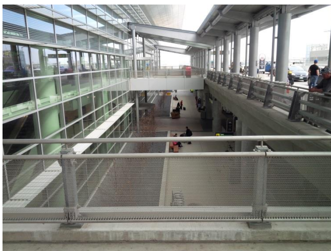
Photo 18: Offset Between Terminal and Bridge Allows Daylight Harvesting
