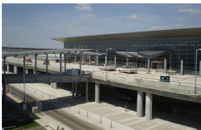
Photo 7: Column Size and Spacing Accommodated Open Structure
