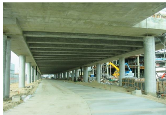
Photo 9: Column Spacing to Provide Large Open Areas on Arrivals Level
