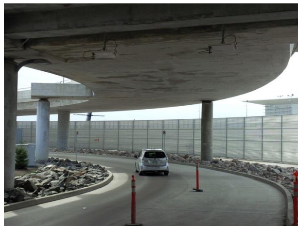
Photo 14: Curved Post-Tensioned Down-Ramp
