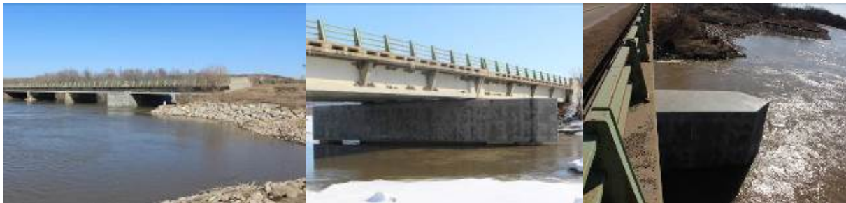
Figure 22 – Completed Pier Foundation
