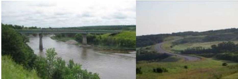
Figure 13 – Existing Bridge on PTH 10 over Souris River
