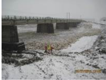
Figure 5 – Completed Bridge Scour Repair Works
