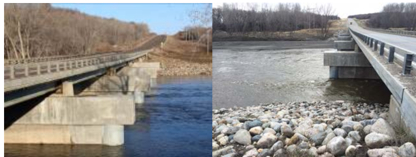
Figure 12 – Completed Pier Modifications and Channel Erosion Protection
