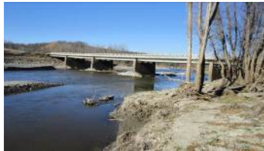
Figure 9 – Existing Bridge on PTH 2 over Souris River Following 2011 Flood
