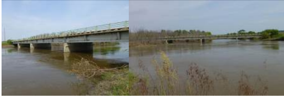
Figure 17 – Existing Bridge on PTH 41 over Assiniboine River
