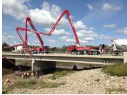
Figure 8– Final Concrete Pour for New SU.5 Pier Footing
