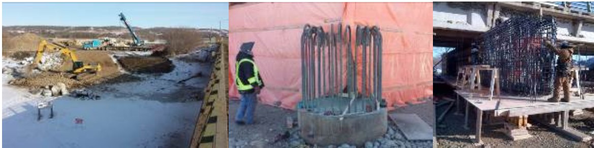
Figure 21 – Work Bridge Construction (left), Completed Caisson (centre), Pier Shaft Reinforcing (right)
