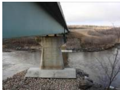
Figure 16 – Completed Pier Foundations
