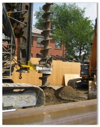
Photo #2 – Pre-augering prior to installing sheetpiles
