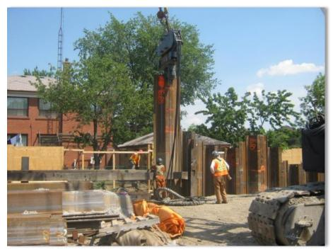
Photo #3 - Installing sheetpiles after pre-augering
