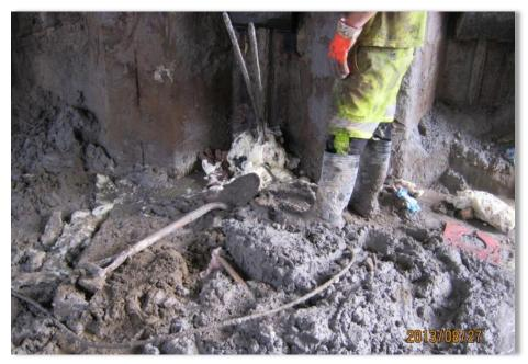
Photo #4 – Foam application to prevent loss of fines
