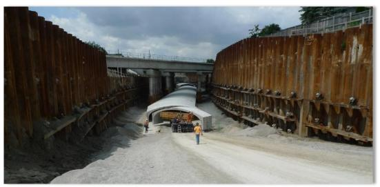
Photo #6 - Completed sheetpiling, subsequent excavation and storm retention tank
