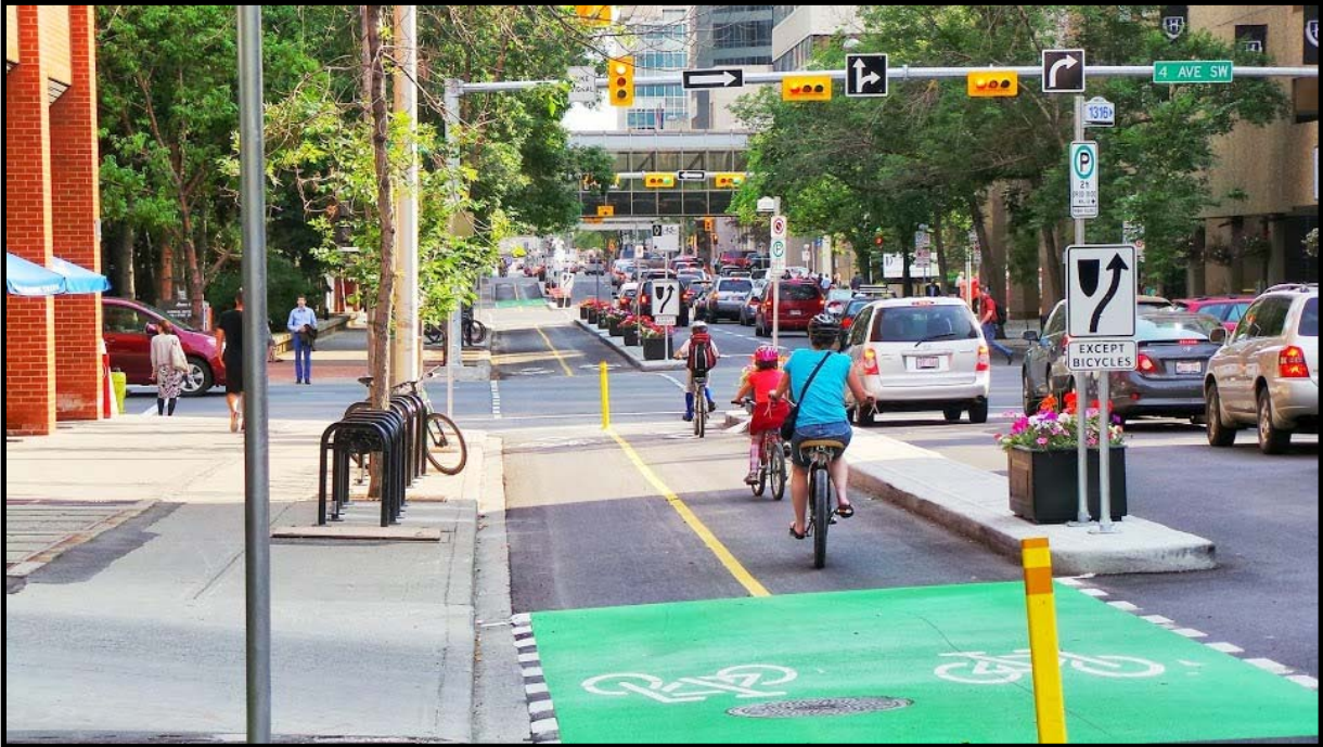
Figure 12: Final product – 7 th Street SW cycle track after opening: Southbound
