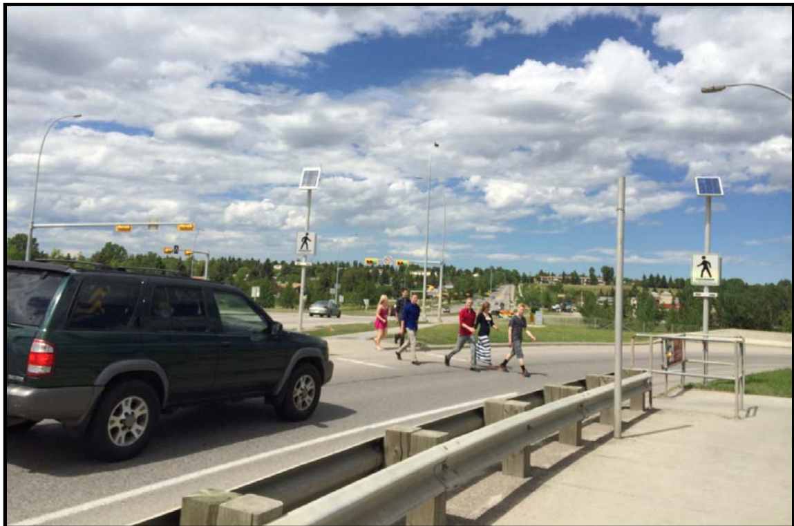
Figure 2: RRFB installed at Glenmore Tr/18 St SE ramp
