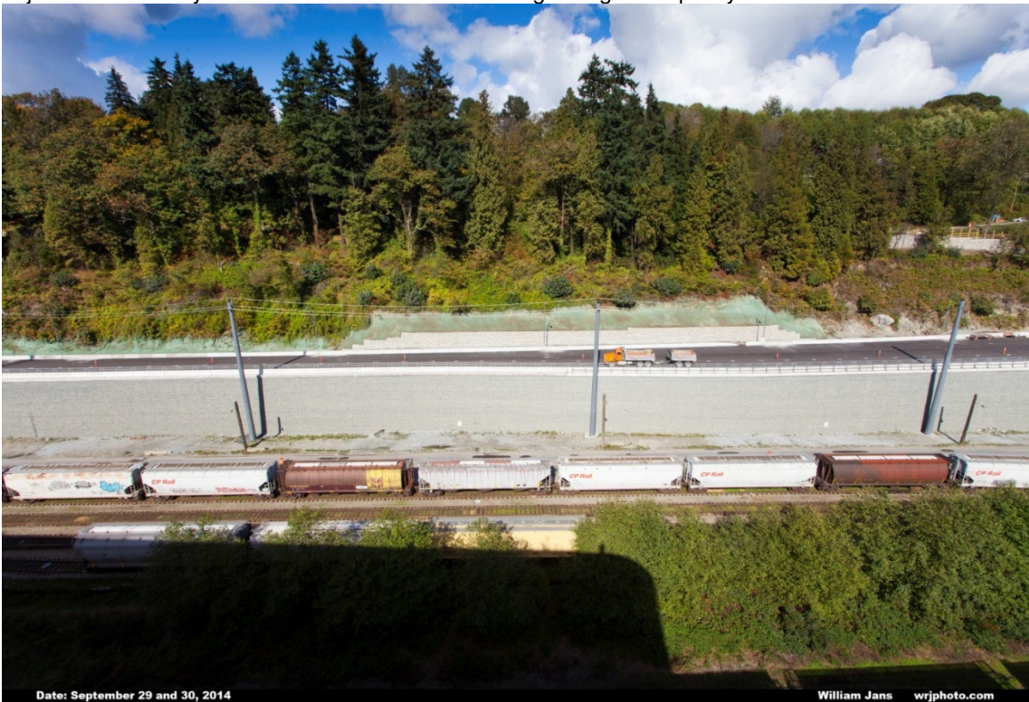
Low Level Road Corridor and Railway, after: Rail improvements along the corridor provide for the future construction of two additional rail tracks parallel to existing tracks to accommodate port growth.
