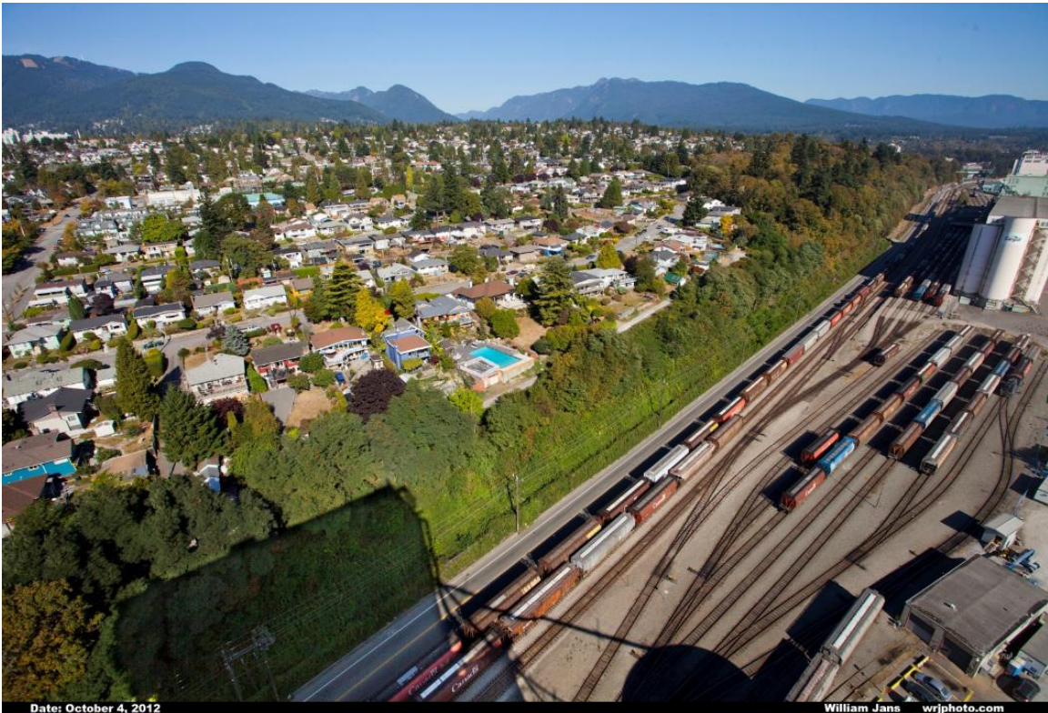
Low Level Road Corridor, before: The laneway and cyclist lane were previously directly adjacent to the rail yard and within the dynamic envelope of moving trains, causing unsafe conditions.
