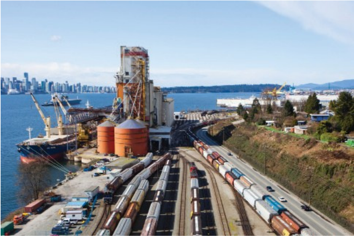
West end, before: The Low Level Road and cyclist lane was previously adjacent to the rail tracks, causing unsafe traffic conditions and noise pollution
