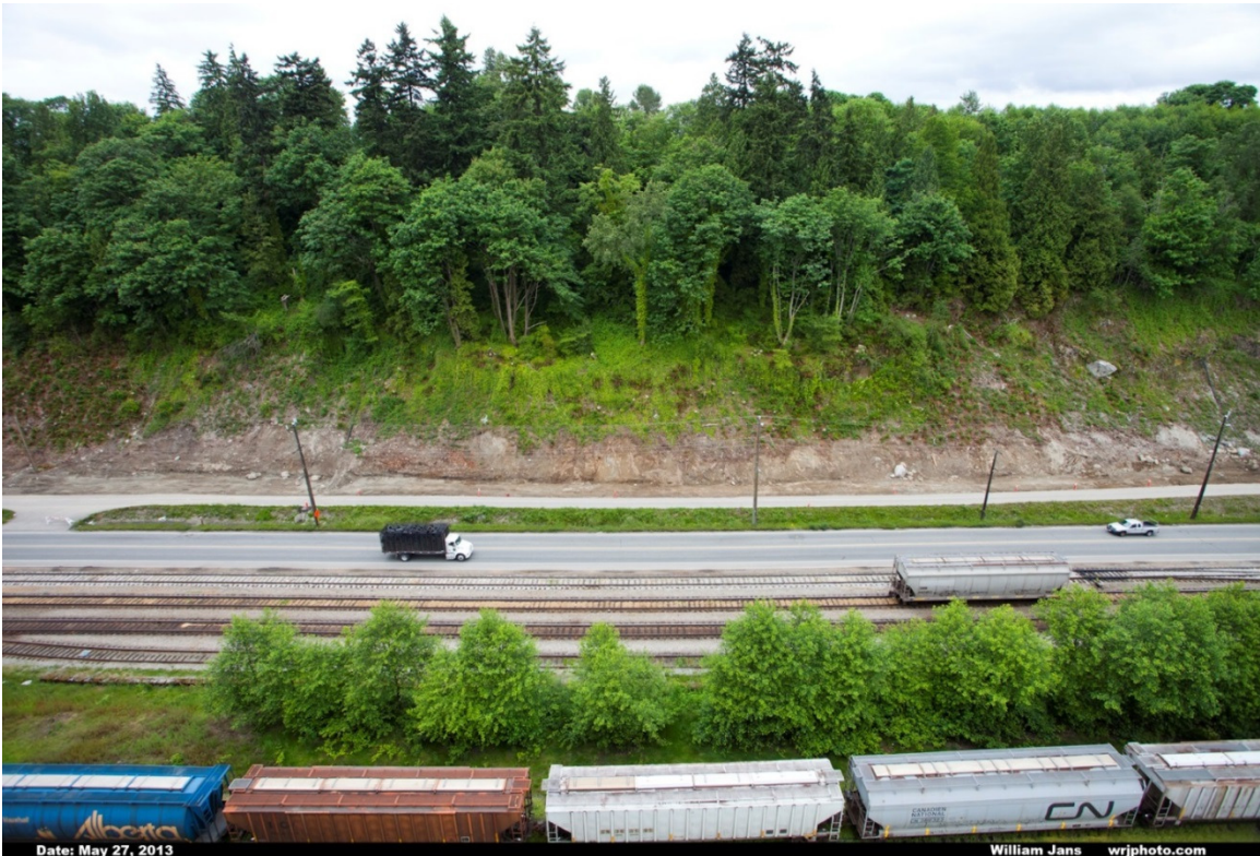
Low Level Road Corridor and Railway, before: Narrow rail envelopes were previously directly adjacent to the rail yard and could not accommodate growing rail capacity demands.
