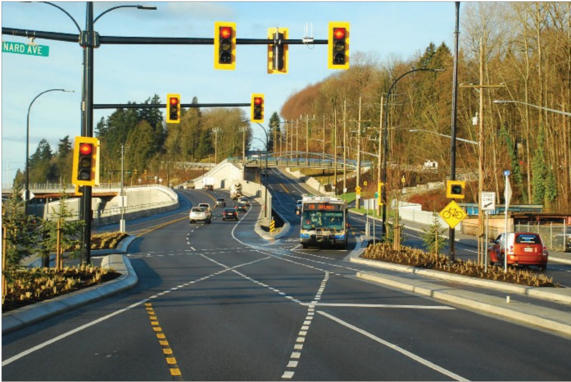
Kennard Avenue Intersection, after: The signalized Kennard intersection efficiently separates traffic along Low Level Road and East 3rd Ave, has fewer merge lanes, and safely accommodates public transit, pedestrians, and bicycle traffic.
