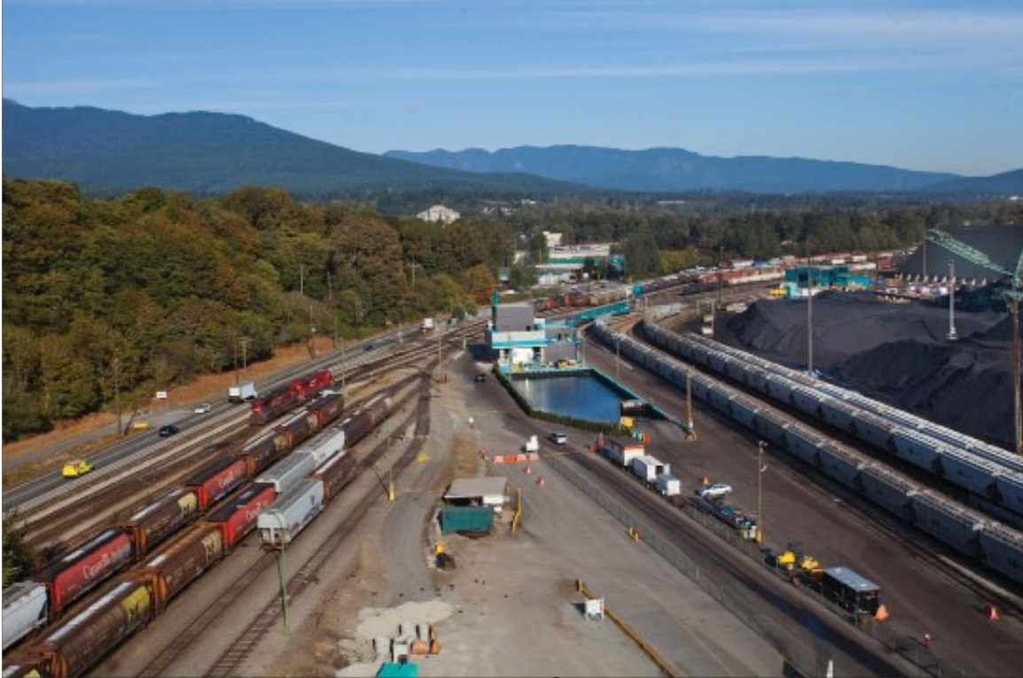
Port access, before: The Neptune and Cargill port terminals were previously accessed by an at-grade rail crossing, causing unsafe and congested traffic conditions
