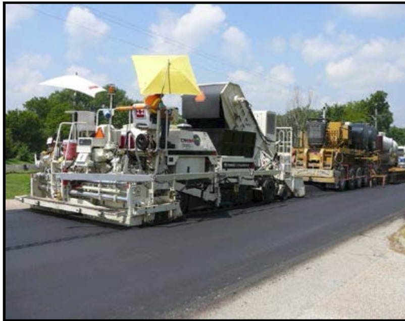
Figure 1-1: Cold In-Place Recycling on Field [5]
