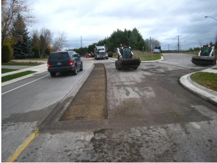
Photograph 10 Repairs of new binder course that incorporated high percentage of RAS.
