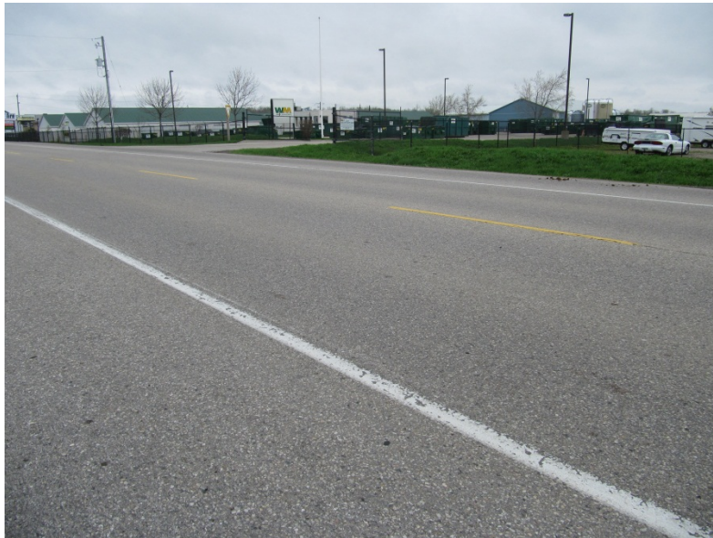
Photograph 2 Good current condition of 10 years old cold in-place recycled pavement.
