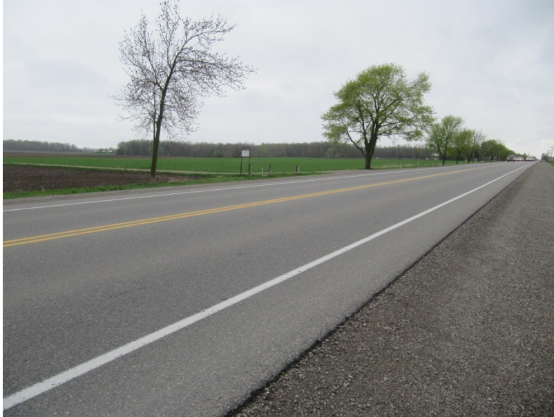
Photograph 5 Excellent current condition of 4 years old foamed asphalt stabilized pavement.
