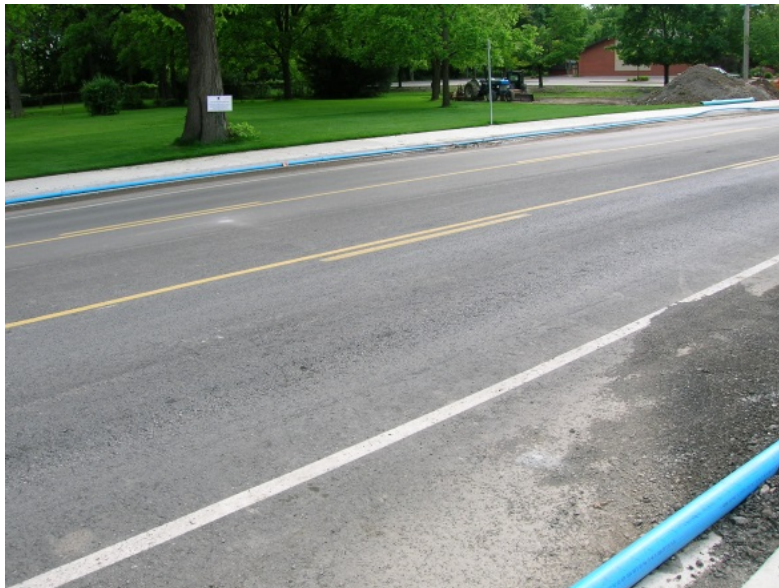
Photograph 7 Raveling of new binder course mix that incorporated very high content of RAP.
