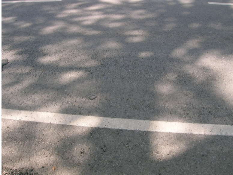
Photograph 6 Microcracking and raveling of new binder course mix that incorporated very high content of RAP.
