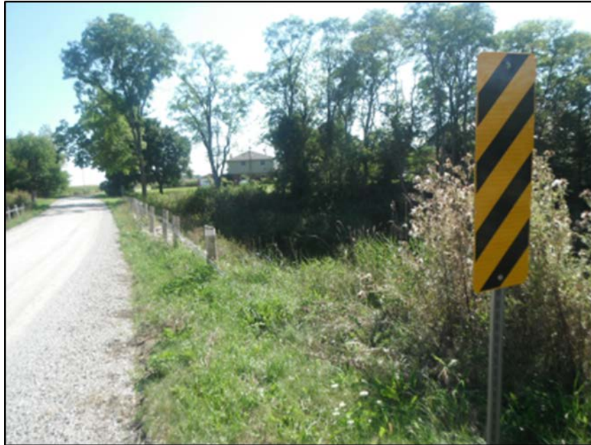
Figure 9 Partially Protected Roadside Hazard
