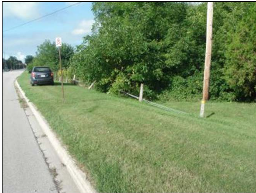
Figure 10 Unnecessary Roadside Safety System
