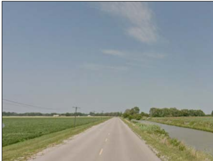
Figure 12 Roadside Drainage Ditch
