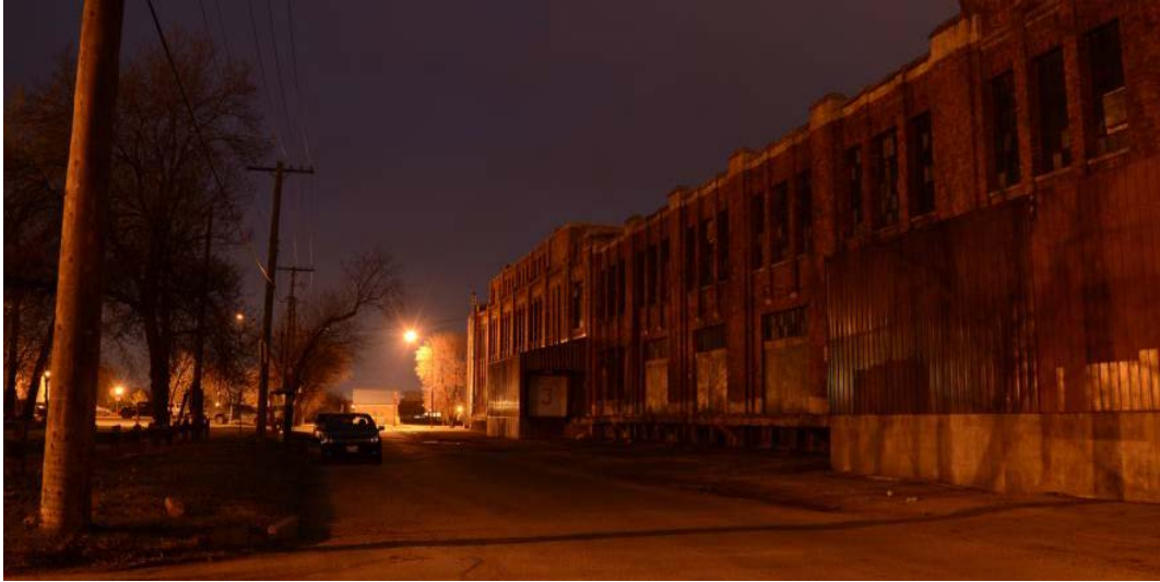
Figure 3: Galt Avenue – Current Conditions
