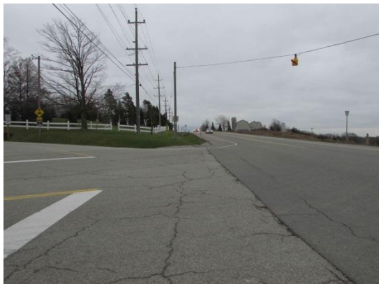
Sawmill Road Looking East
