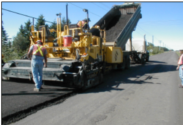
Figure 6 - Placement of 20mm Corrective Aggregate with ABG Paver, Ellerslie Road
