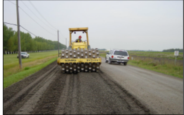
Figure 10b - Vibratory Pad Foot Ellerslie Road
