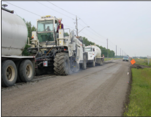
Figure 9a - Recycling Train Ellerslie Road
