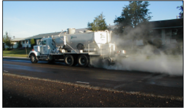
Figure 8b - Spreading Cement on Surface of 150 Avenue
