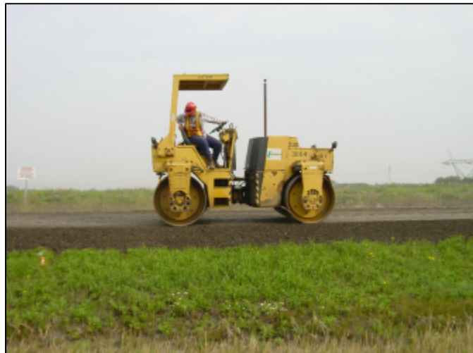
Figure 12 - Final Compaction Ellerslie Road
