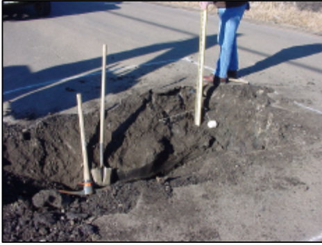
Figure 5a - Test Pit on Ellerslie
