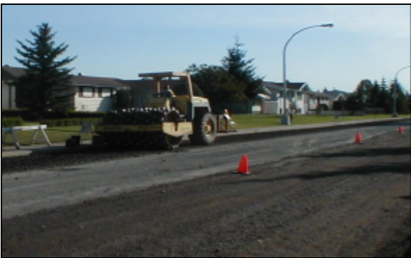
Figure 10a - Vibratory Pad Foot 150 Avenue
