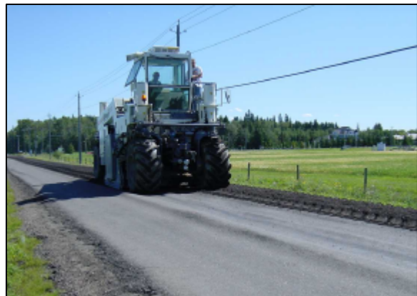
Figure 7 - Pre-pulverization of Heavily Rutted Section of Ellerslie Road
