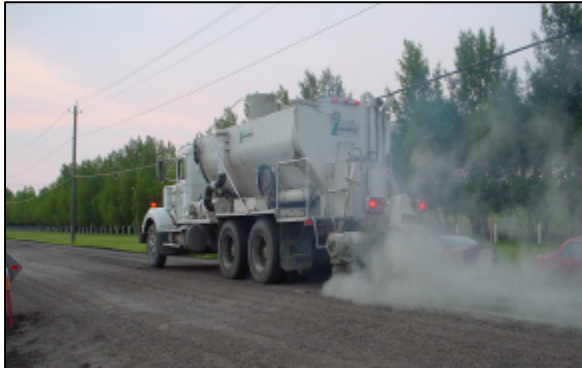
Figure 8a - Spreading of Cement on the Surface of Compacted Aggregate Ellerslie
