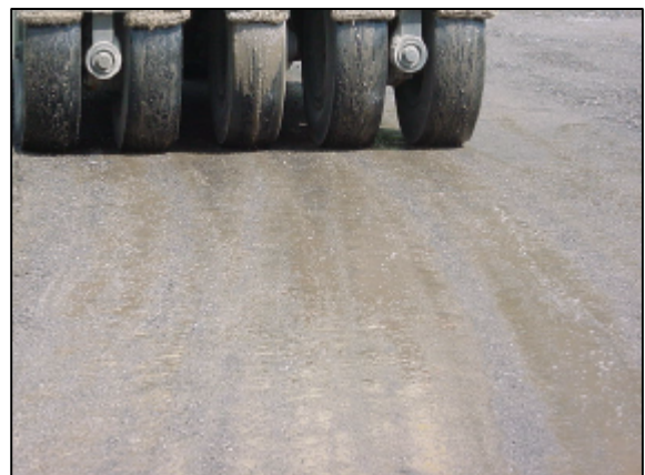
Figure 14 - Slushing with Pneumatic Roller
