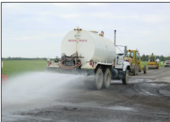
Figure 13 - Watering of Surface Ellerslie Road
