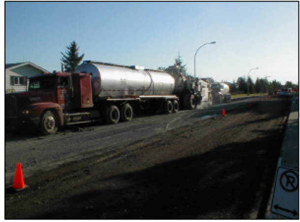
Figure 9b - Recycling Train 150 Avenue
