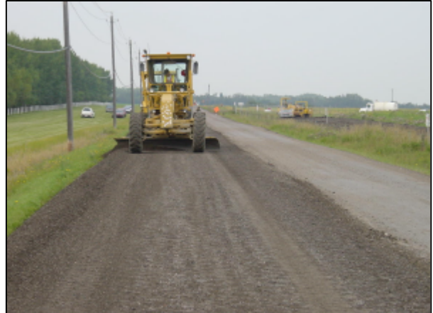
Figure 11b - Grading Ellerslie Road
