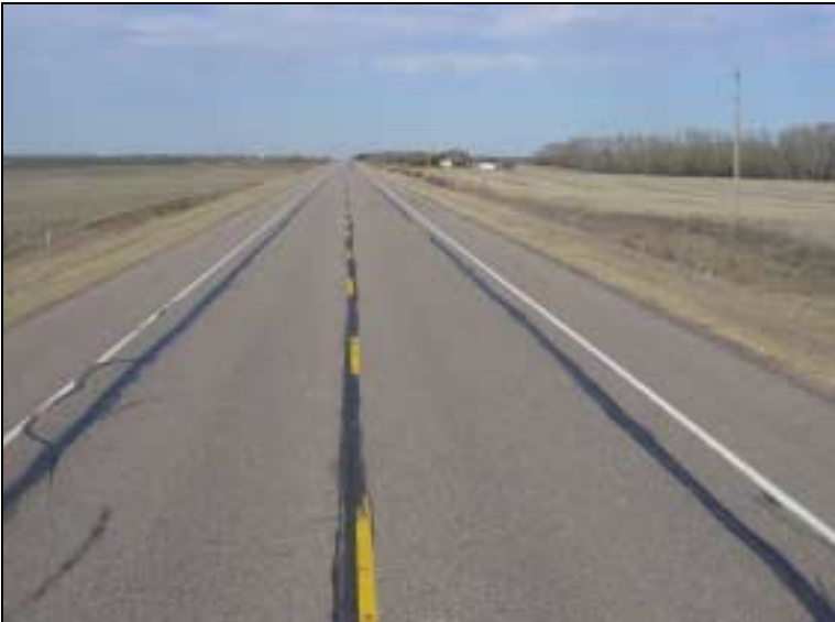
Figure 10 – Test Section 7, 200-300A, 4 cracks/km
