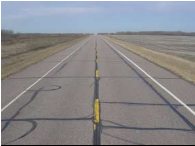
Figure 4 – Test Section 1, 80-100B, 143 cracks/km
