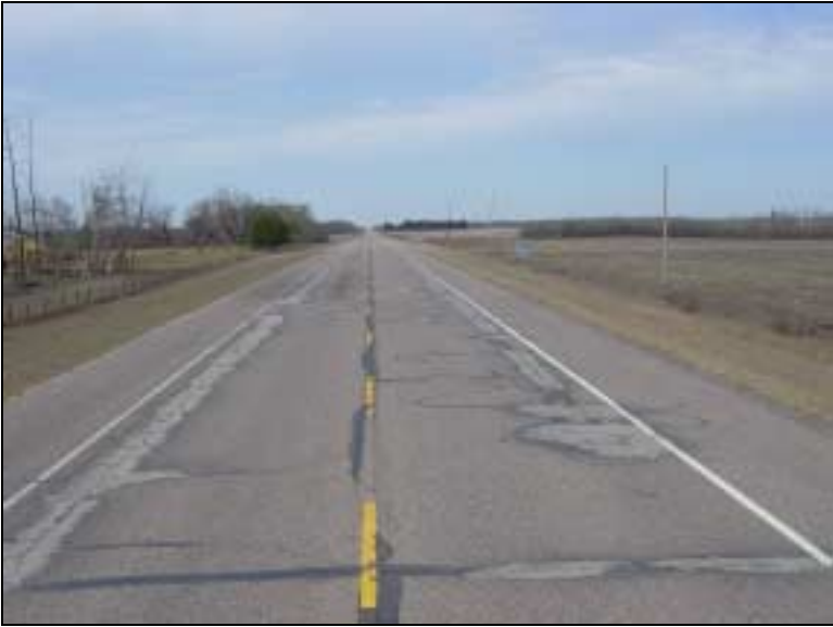
Figure 8 – Test Section 5, 80-100A, 119 cracks/km
