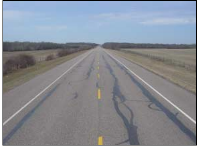
Figure 9 – Test Section 6, 150-200A, 37 cracks/km
