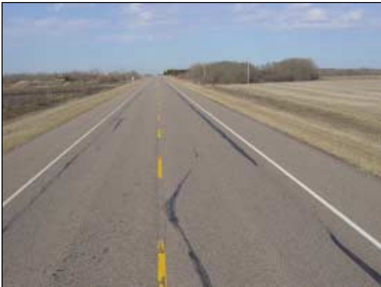
Figure 6 – Test Section 3, 300-400A, 0 cracks/km
