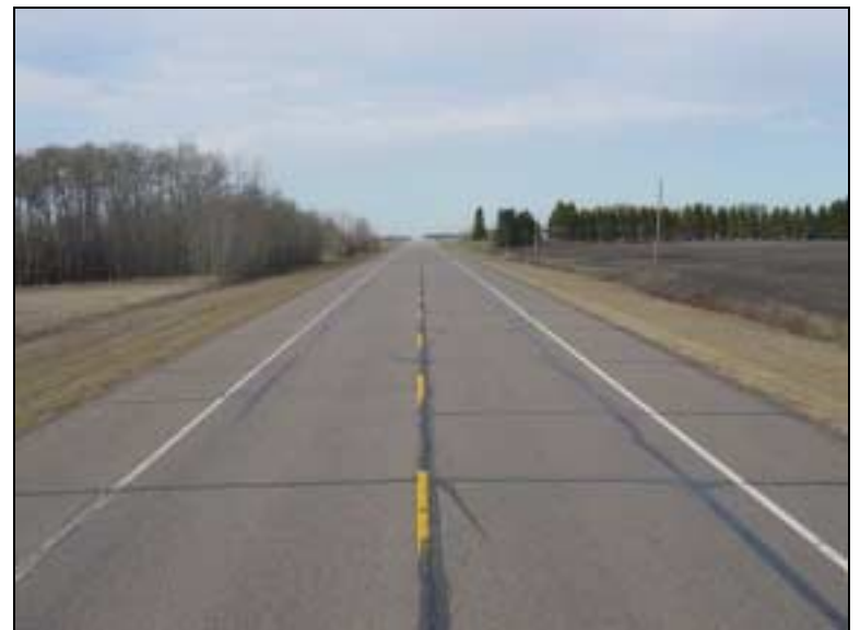
Figure 7 – Test Section 2, 80-100C, 163 cracks/km
