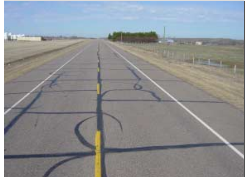
Figure 5 – Test Section 2, 150-200B, 180 cracks/km
