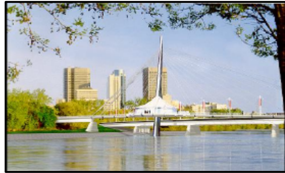
Figure 1: Provencher Pedestrian Bridge
