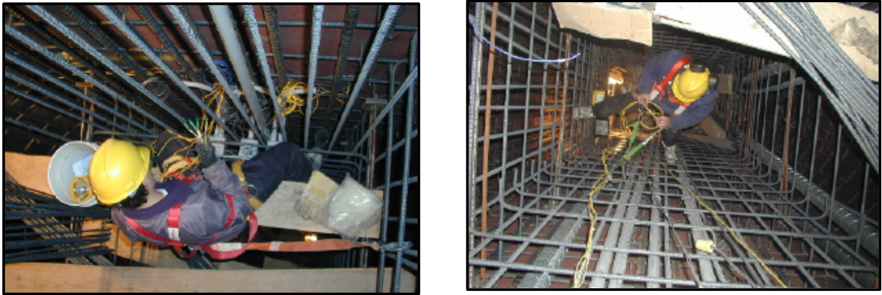
Figure 10: Wiring the sensors to the junction box before concrete pour
