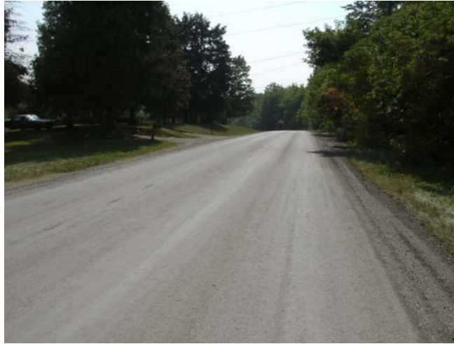
Figure 5. Final Pavement Surface Prior to HMA Overlay.
