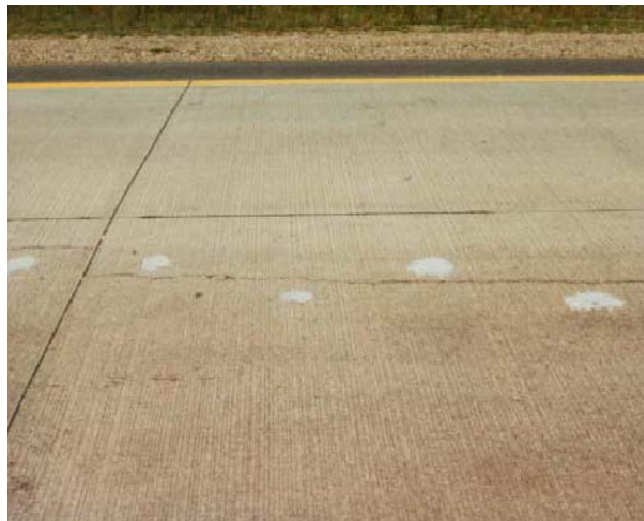
Figure 9. Load transfer restoration using slab stitching.
