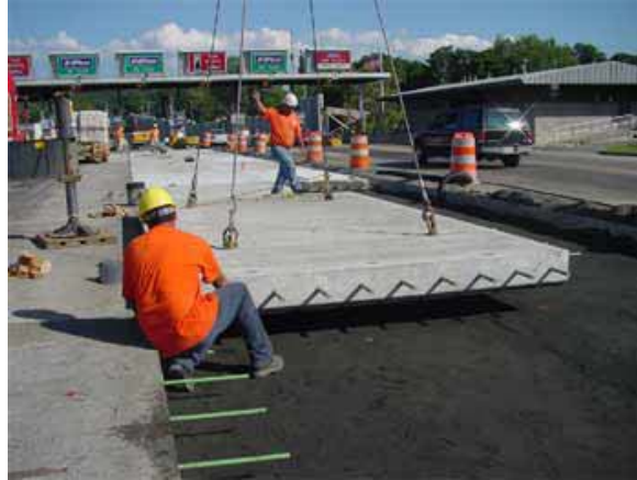
Figure 10. Fort Miller precast concrete slab placement technique.
