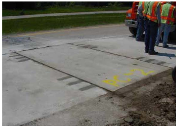
Figure 11. Completed pre-cast slab repair.
