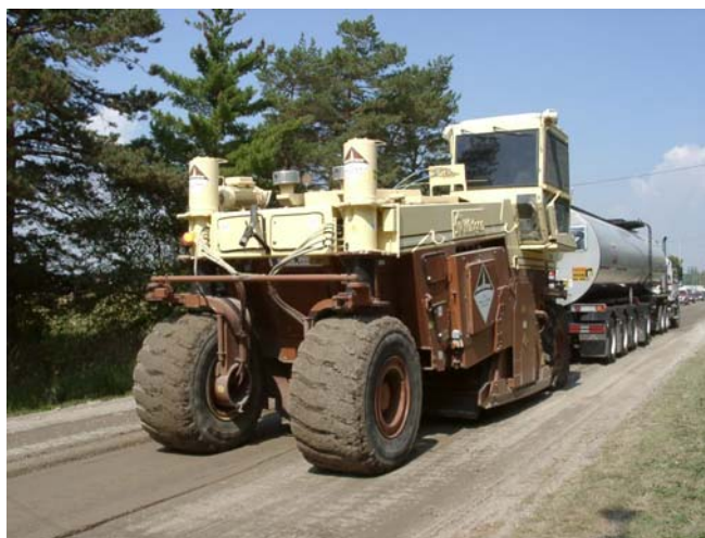
Figure 4. Foamed Asphalt Recycling Train.
