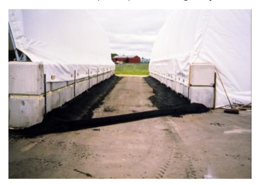
2). Asphalt curbing around asphalt pad with gap at low point for water to drain into buried storage tank (white tank lid visible in centre of photo).
