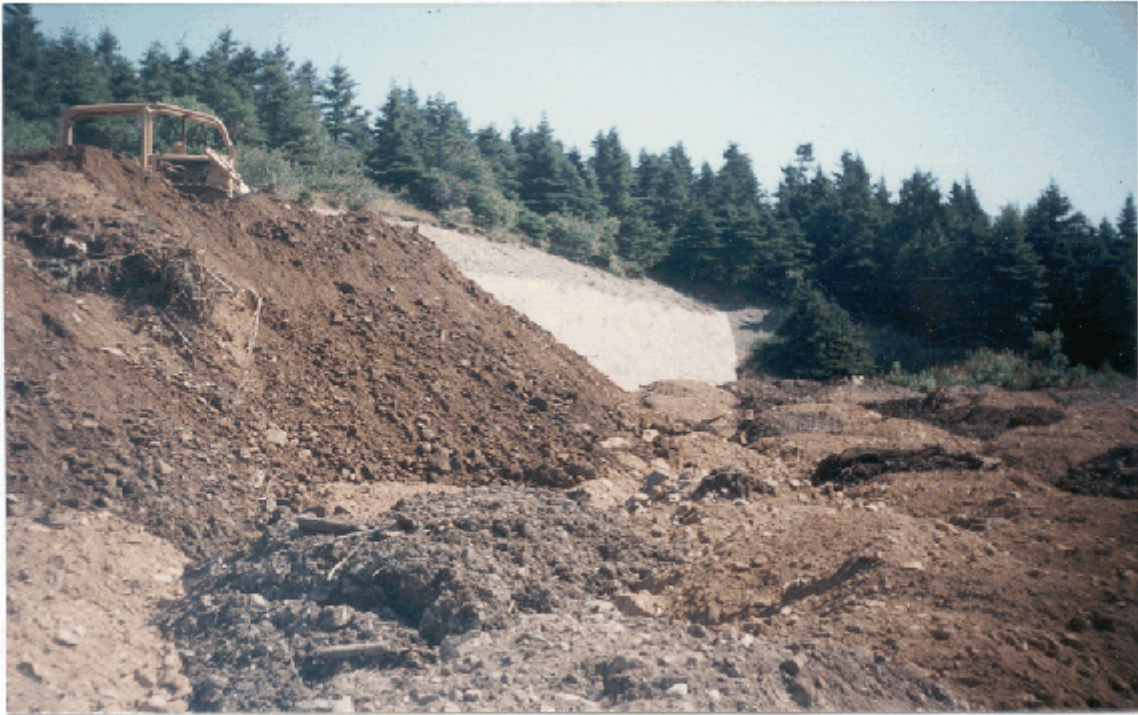
USM being placed in an abandoned pit near Oxen Pond Road to cover up graffiti rock face and re-establish original grades.
