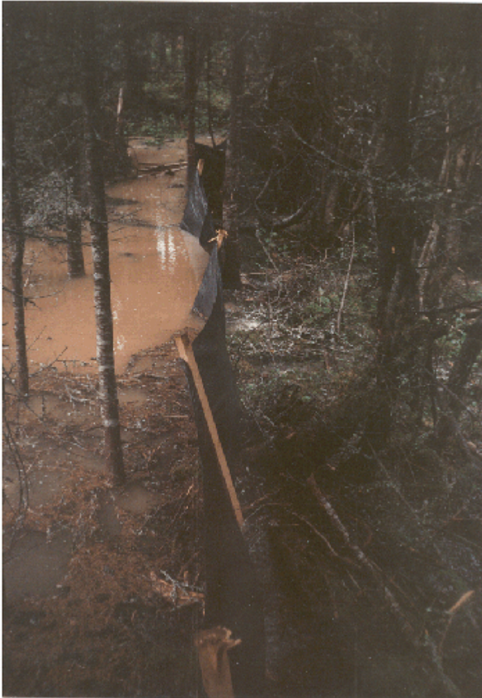
Surface runoff confined. Equipment operating "in the dry".
