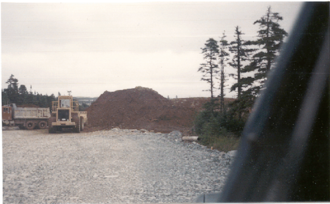
Topsoil saved where encountered. Being loaded and hauled to storage site.
