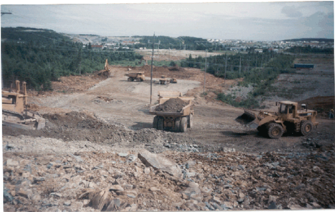
Extensive mobilization of heavy equipment, grubbing, topsoil stripping, USM & OM removal.
