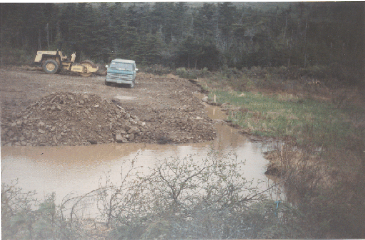
Silted water confined to construction zone in area of high ground water. Grubbing and infilling proceeding simultaneously.
