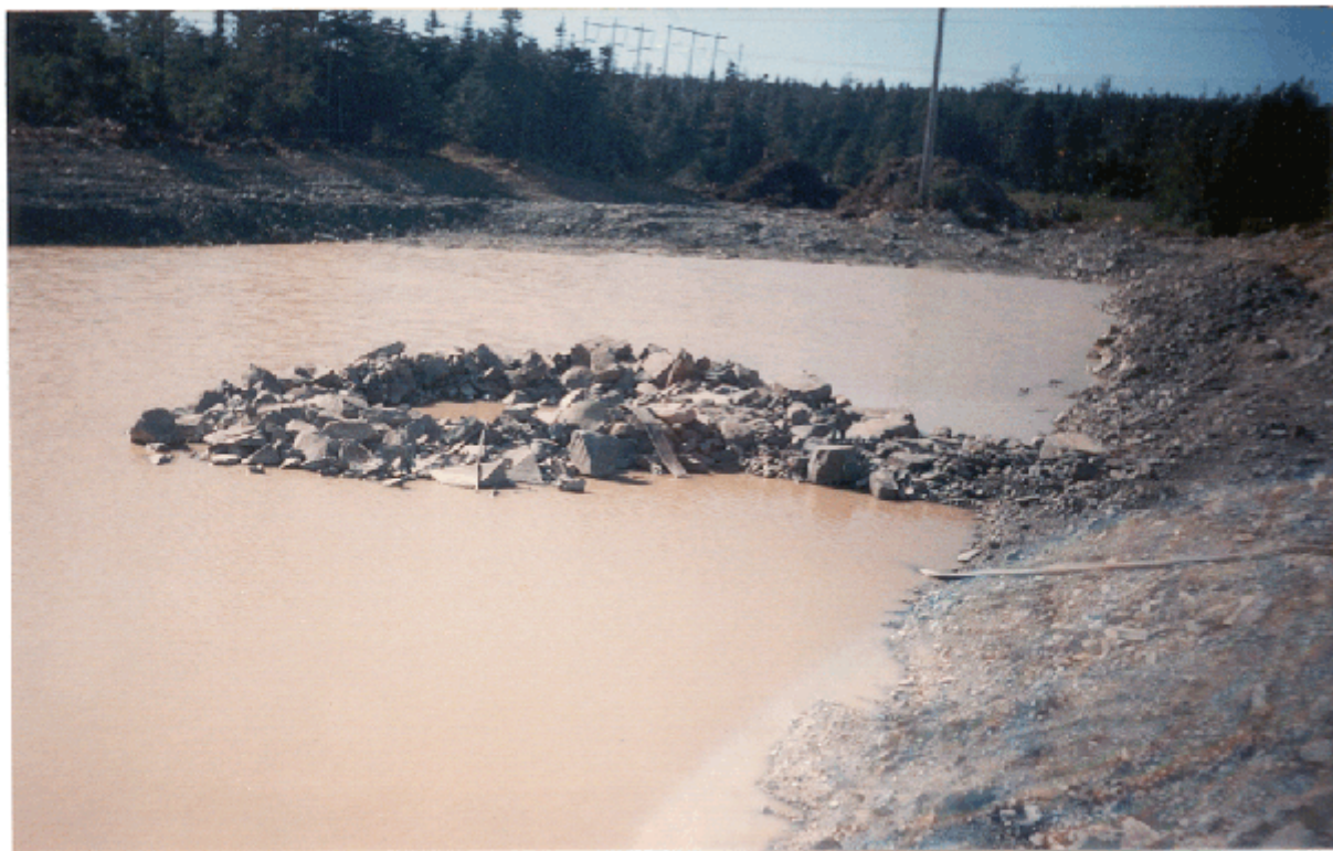
Large settling basin provided to contain and settle out silted water prior to release.
