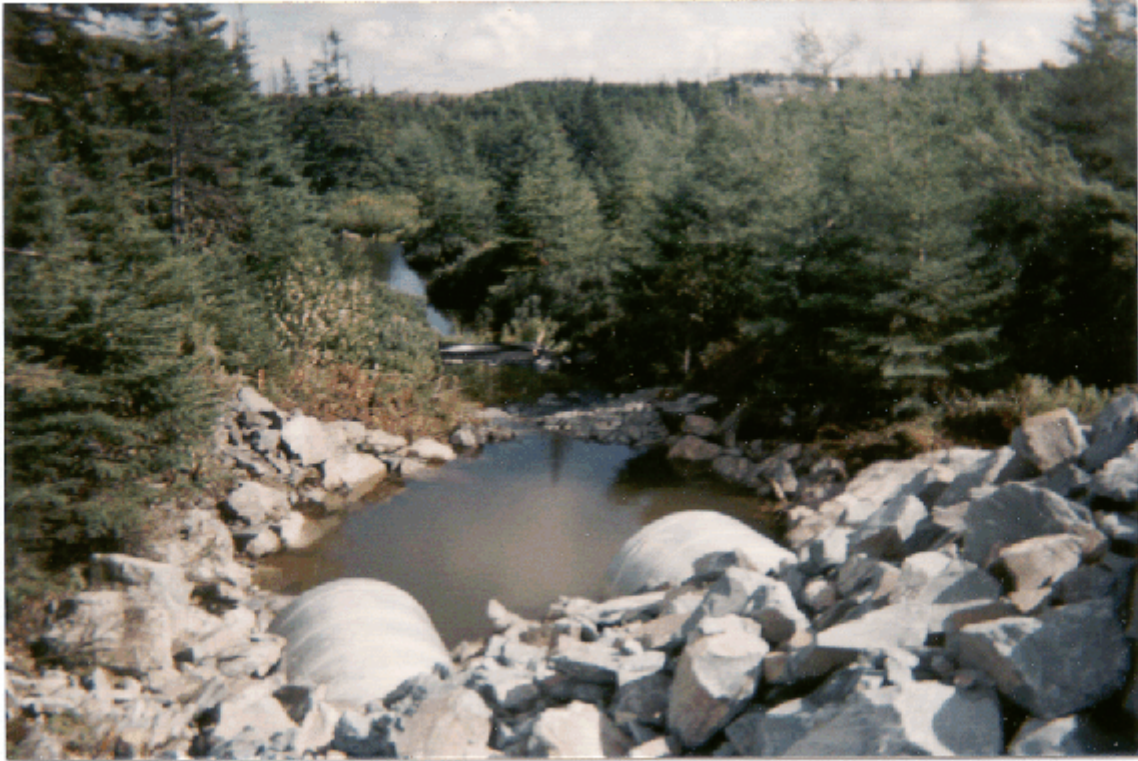
Large pools constructed at all culvert outlets Bremigan's Pond Brook.
