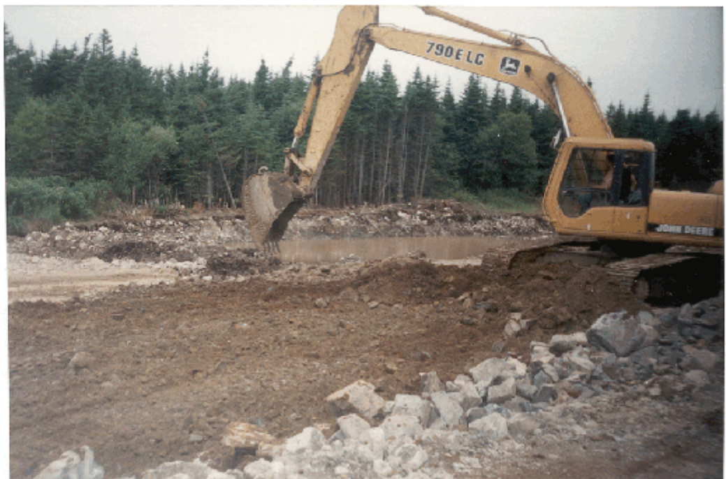
Surface runoff confined. Equipment operating "in the dry".
