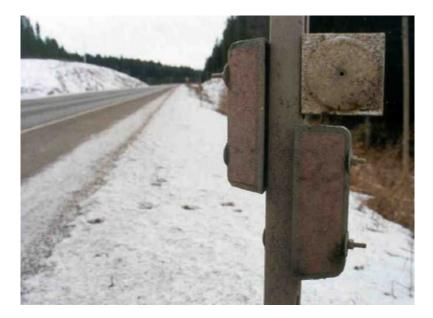
Figure 8. Wildlife warning reflectors subjected to winter roadside conditions
