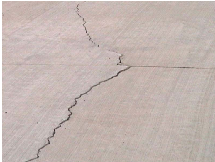
Figure 3. Crack from frost heave with characteristic difference in slab surface.
