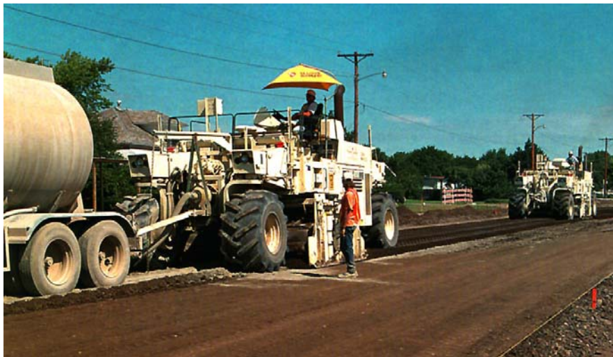
Figure 5. Soil stabilization can improve the soil's properties for both construction and pavement performance, including frost action.
