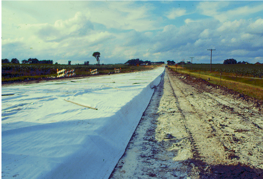
Figure 6. Insulating blankets in place on freshly-placed concrete slab.
