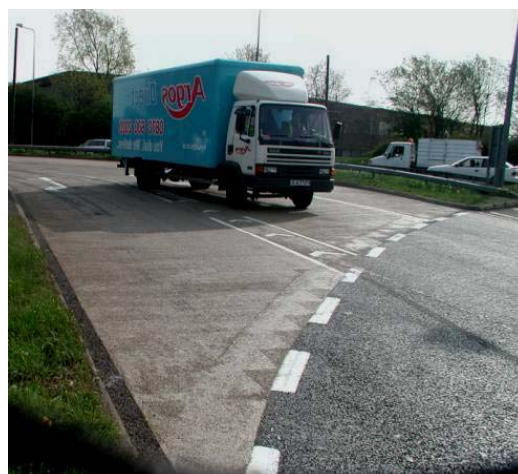
Figure 16 - Shell-coat Skid Treatment
