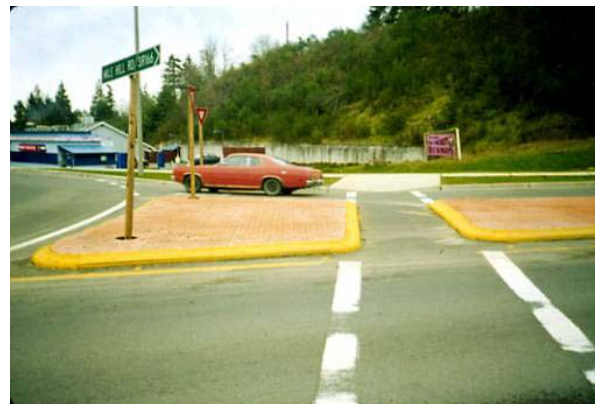
Figure 11 - Cross Walk Alignment That Is Too Enticing
