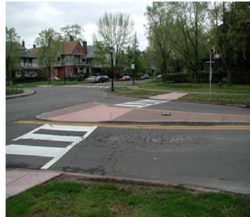
Figure 9 - Poorly Located Cross Walk
