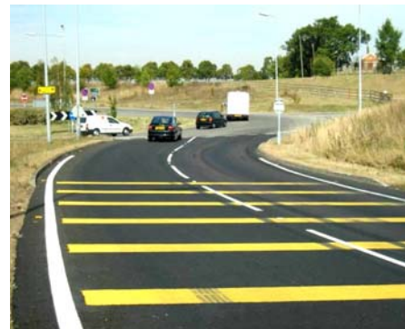
Figure 13 - Bar Markings for Rural Conditions
