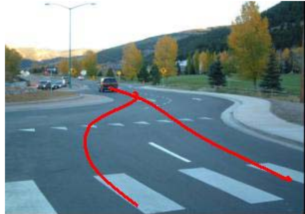
Figure 3 - Insufficient Entry Path Curvature (This layout also suffers from entry path overlap)
